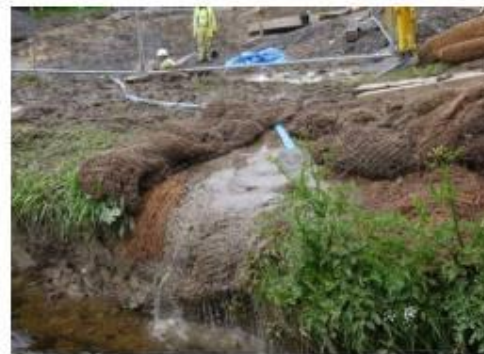
Deployed to treat muddy excavation water
