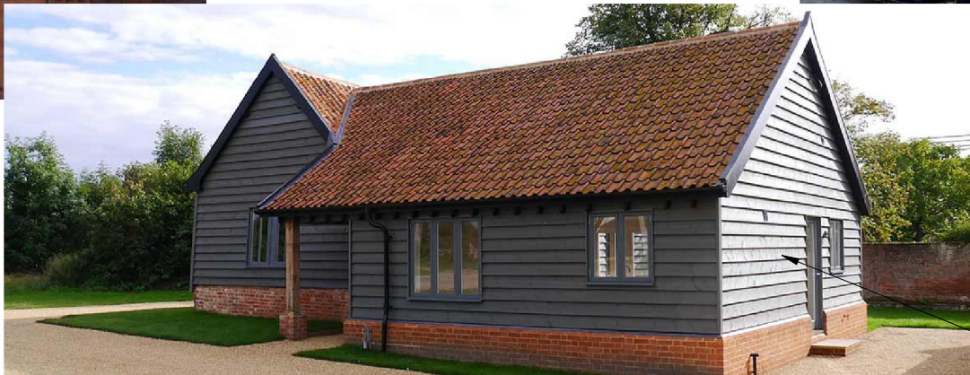
Cement Fibre board is no-maintenance and allows easy build-over on existing walls, whilst giving a rural look
