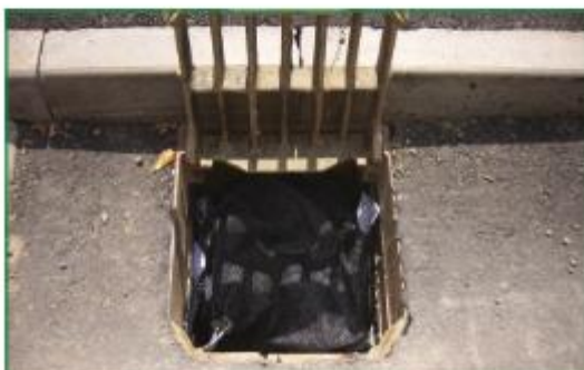
5. Close gully grid.
