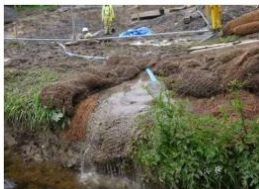
Deployed to treat muddy excavation water
