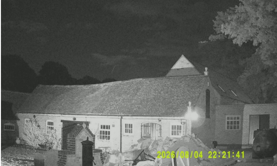
Figure 23 Position 1 darkest point – southwestern elevations of B2 and B2
