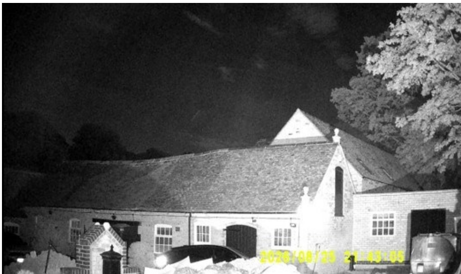
Figure 26 Position 1 darkest point - southwestern elevations of B2 and B2
