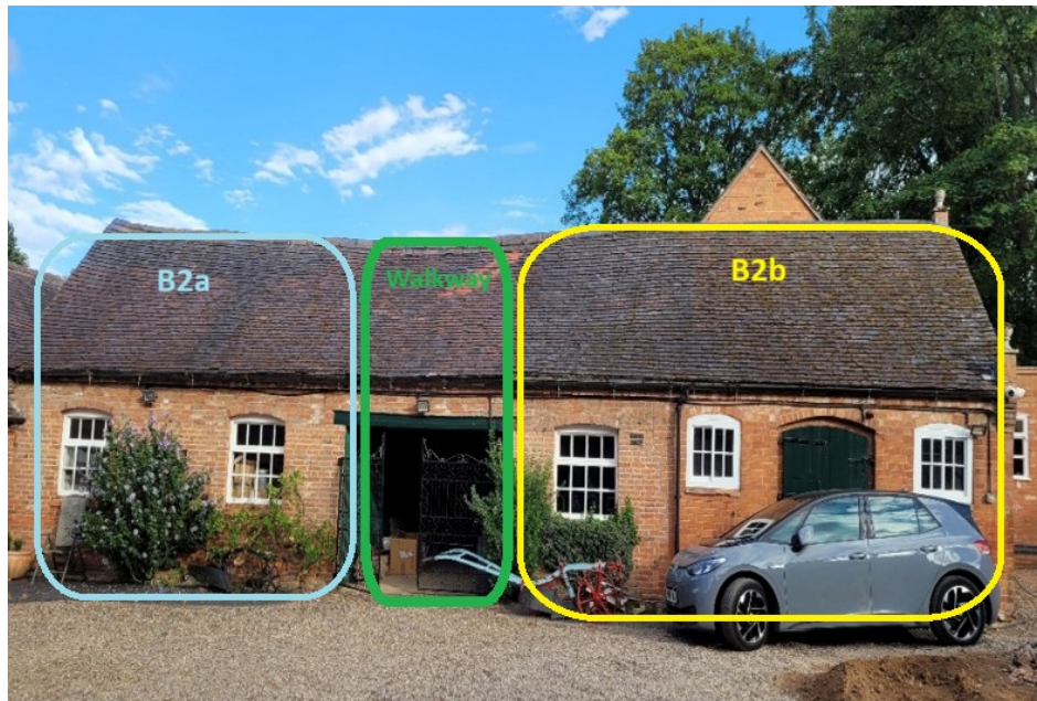
Figure 10 B2 northern facing elevation showing separate B2a and B2b areas and walkway (green) leading to rear of building and connecting the two separate rooms.
