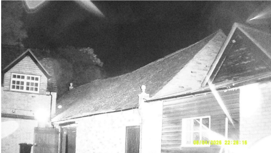
Figure 25 Position 3 darkest point – northern and northeastern facing elevations B2
