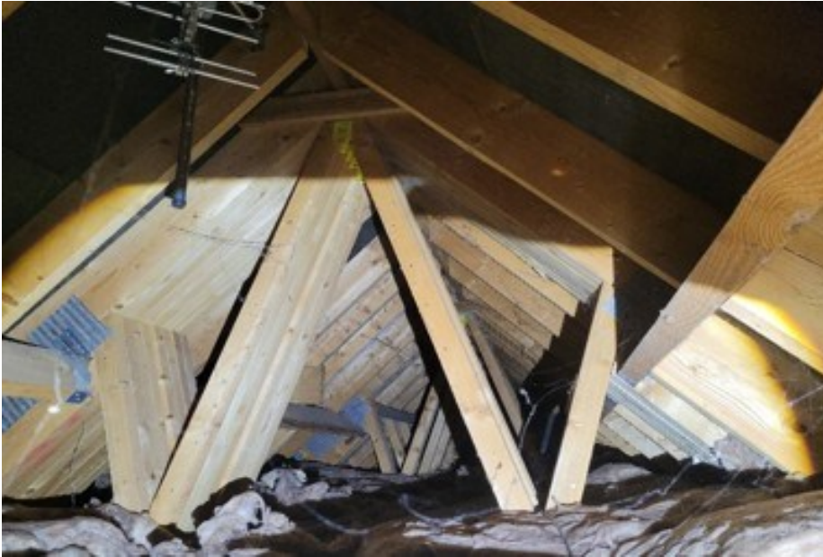
Figure 8 B1 roof void
