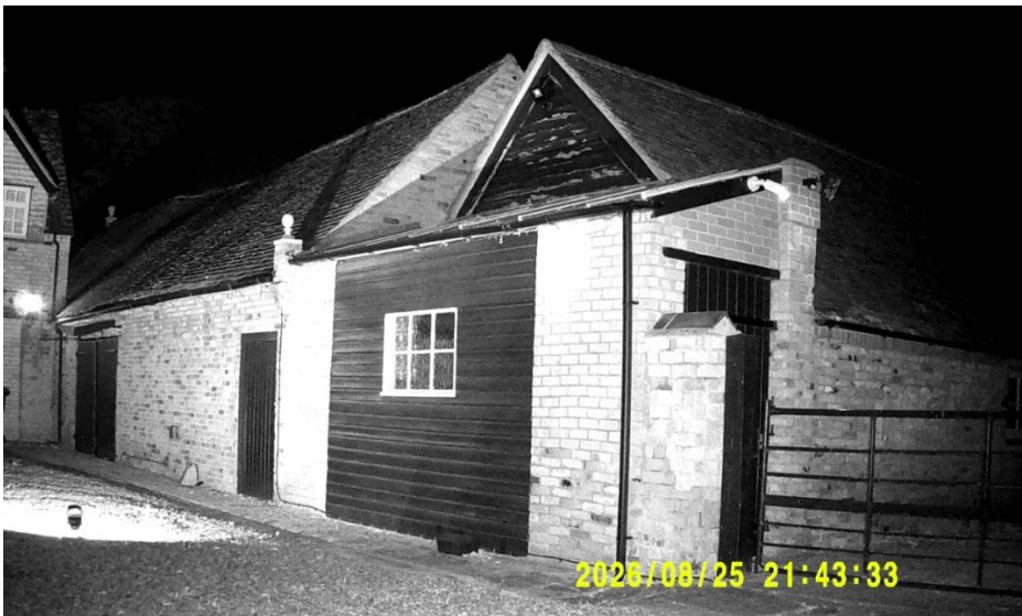
Figure 28 Position 3 darkest point - northern and northeastern facing elevations B2
