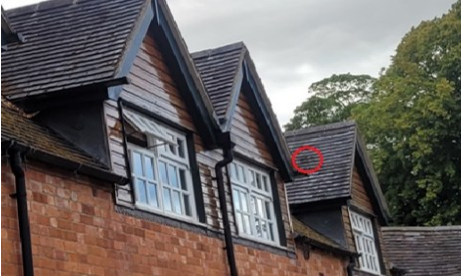
Figure 5 Lifted tile dormer window facing south
