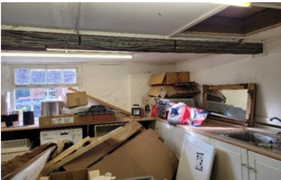
Figure 14 B2a open room showing loft location
