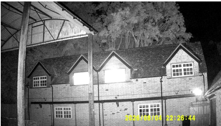
Figure 24 Position 2 darkest point – northern facing elevation of B1
