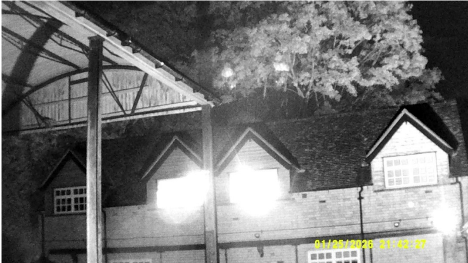
Figure 27 Position 2 darkest point - northern facing elevation of B1
