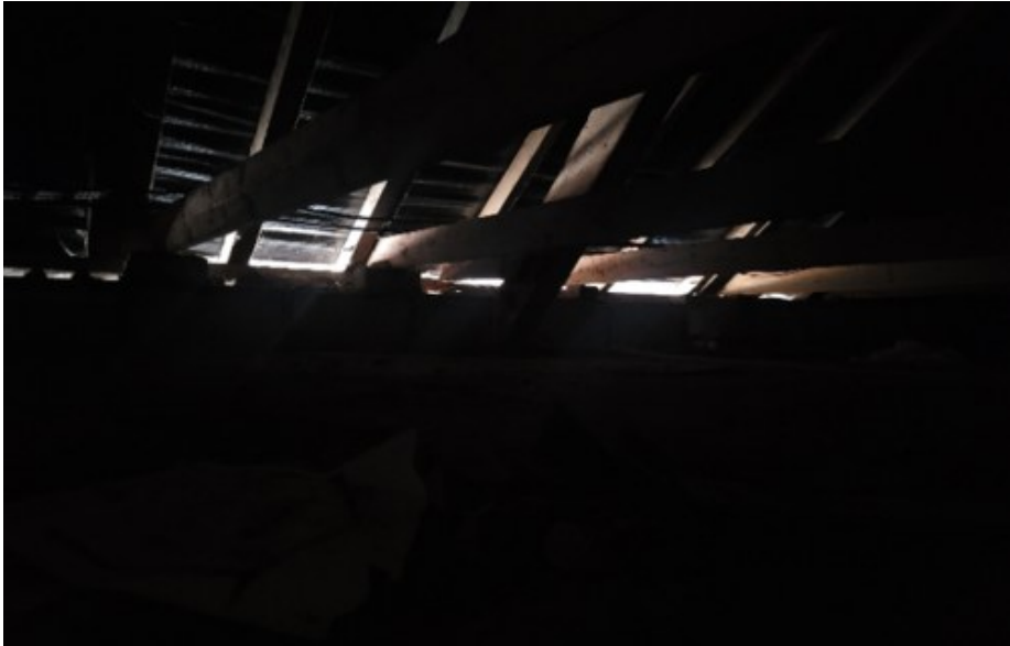
Figure 18 Light ingress through roof into B2a loft
