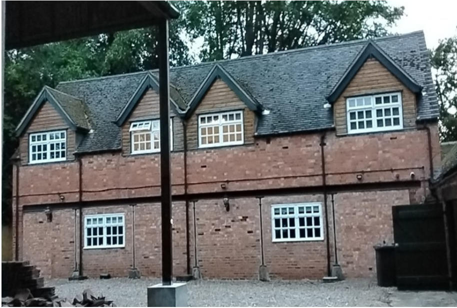
Figure 3 Building 1 northeastern facing elevation
