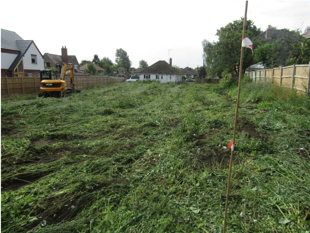
Figure 4: Removing vegetation. Looking north
