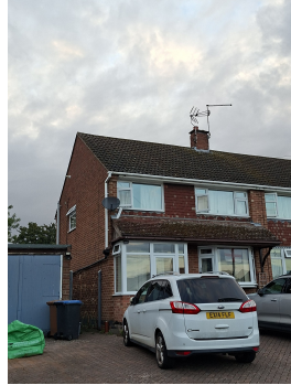
V2 B1-1 surveyor photo
