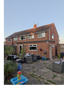
V1 B1-2 surveyor photo
