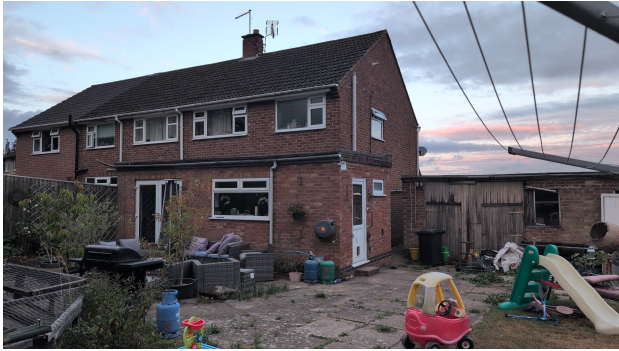
V2 B1-2 surveyor photo
