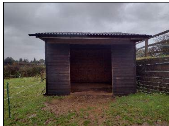
Photograph 25: Field Shelter 'B4'
