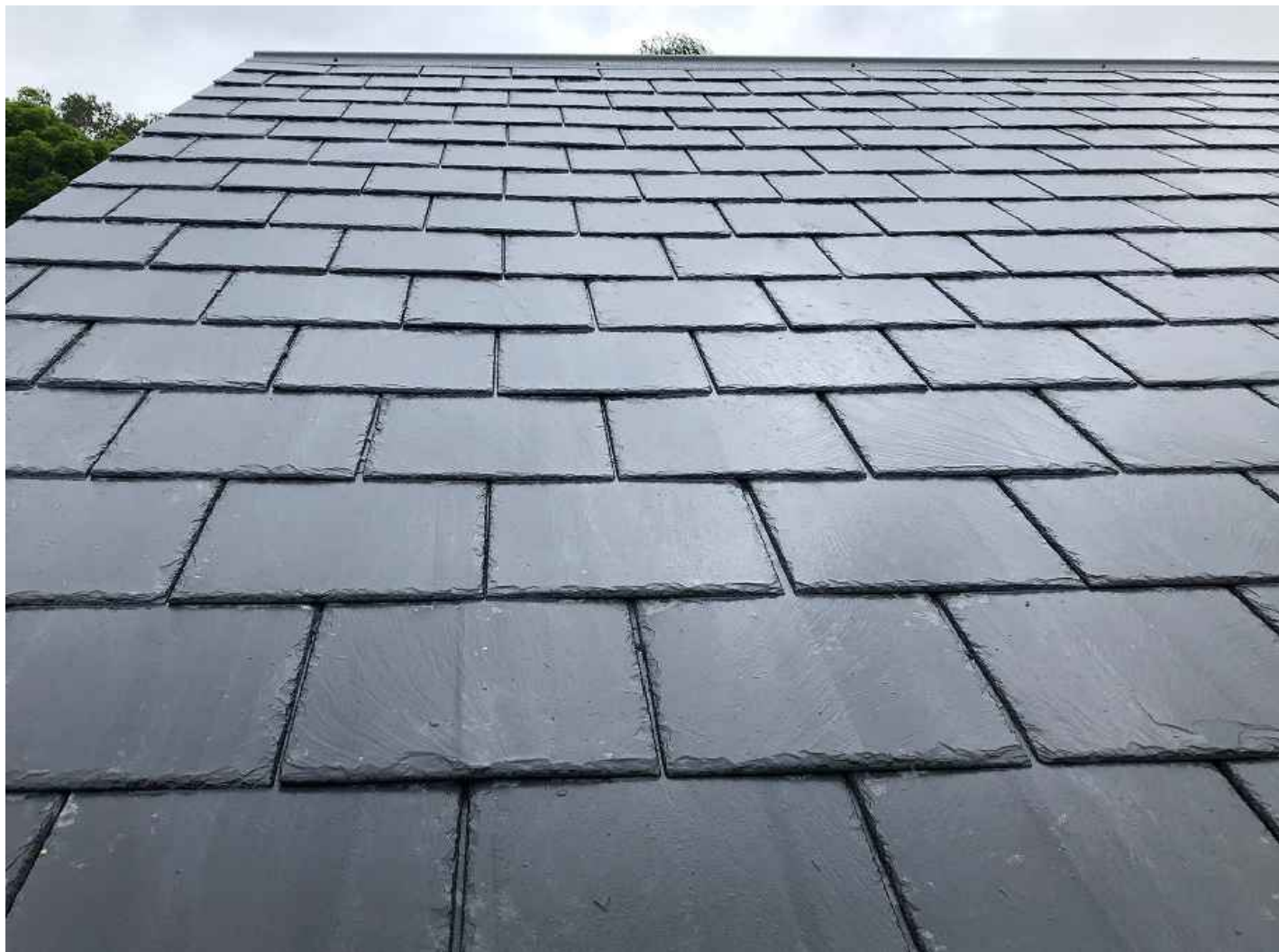
Example Roof Covering
