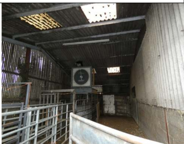
Photograph 59. The interior of Barn 17
