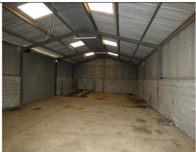
Photograph 48. The interior of Barn 3
