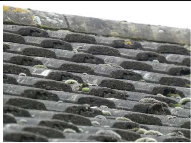
Photograph 10. Example of the interlocking concrete tiles on the gable projections to the north-east of the Farmhouse
