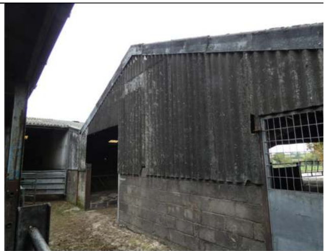
Photograph 52. The north-east elevation of Barn 6 and Barn 7
