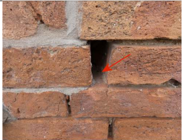
Photograph 38. Single bat dropping in a crevice in the brickwork on the north-east side of The Granary
