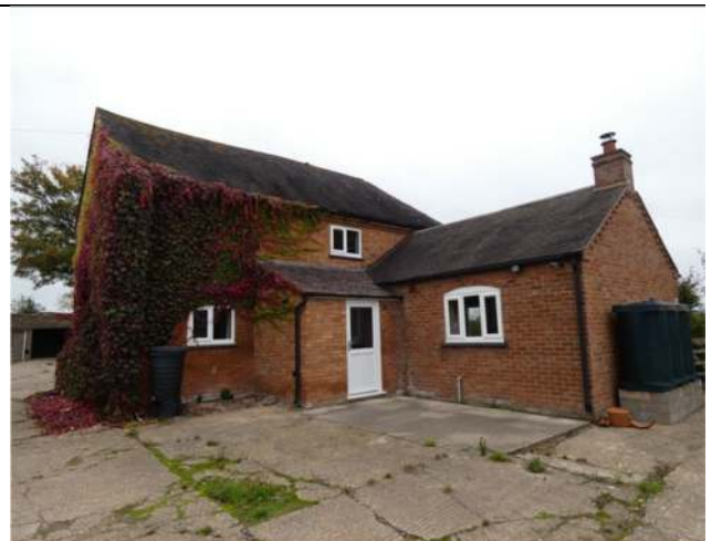
Photograph 30. The south-west and south-east elevations of The Granary
