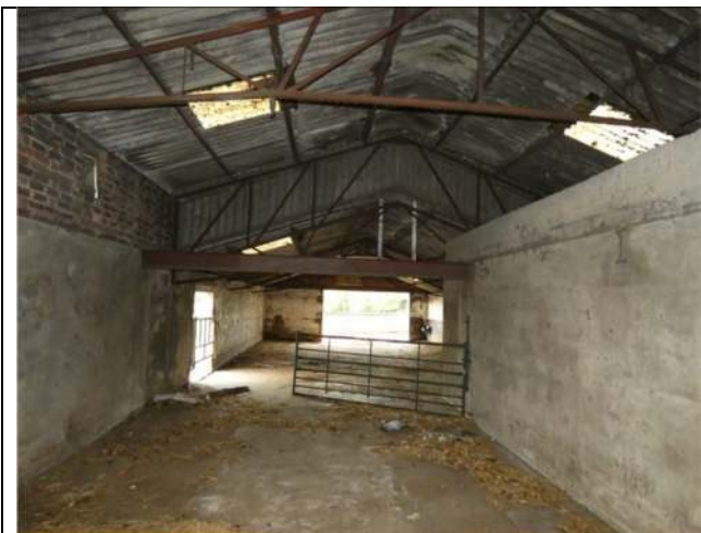
Photograph 53. The interior of Barn 5 (view to south-west)
