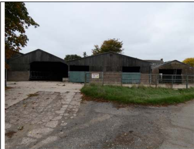
Photograph 51. The south-west elevations of Barns 5-7
