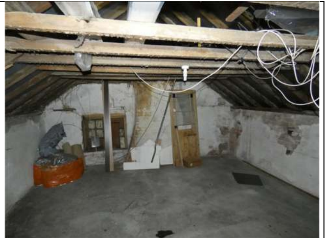
Photograph 22. The attic room in the south-east half of the main part of the Farmhouse (view to south-east)
