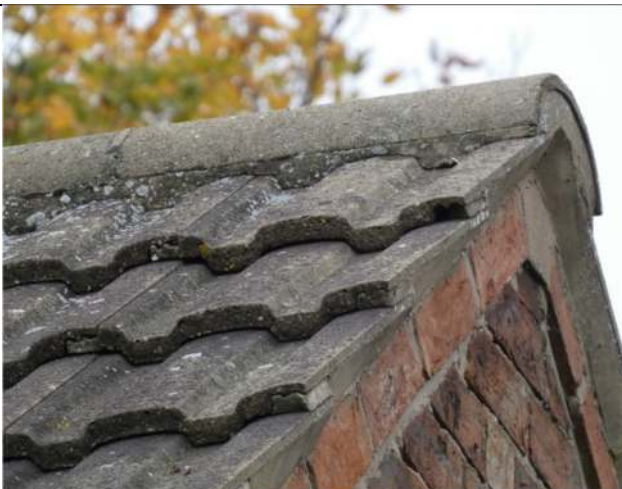
Photograph 11. Further example of the interlocking concrete tiles on the gable projections to the north-east of the Farmhouse
