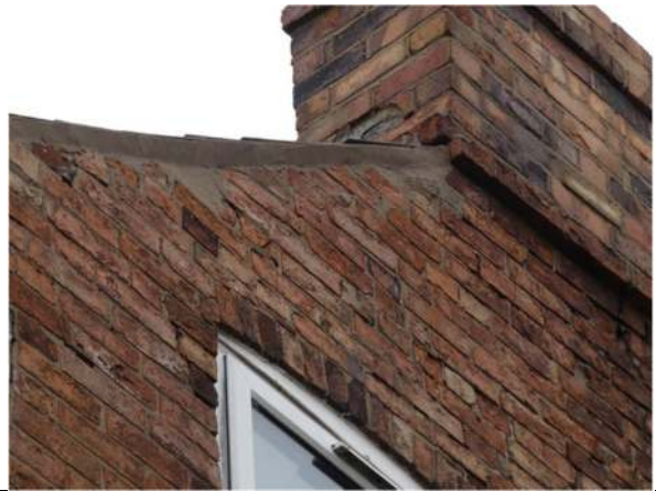
Photograph 8. Example of the roof edge on the main part of the Farmhouse
