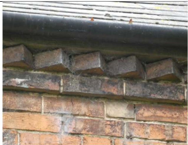
Photograph 16. Example of the corbelling on the Farmhouse
