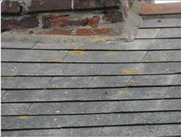
Photograph 7. Example of the slates on the south-west facing roof pitch of the main part of the Farmhouse
