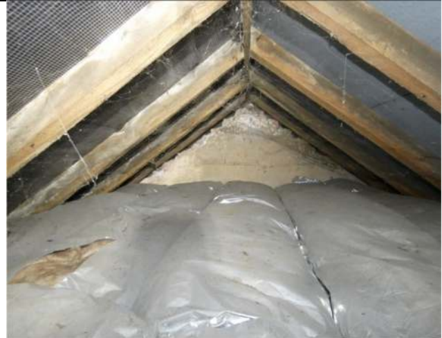
Photograph 20. The section enclosed roof void in the south-east half of the main part of the Farmhouse (view to north-west)
