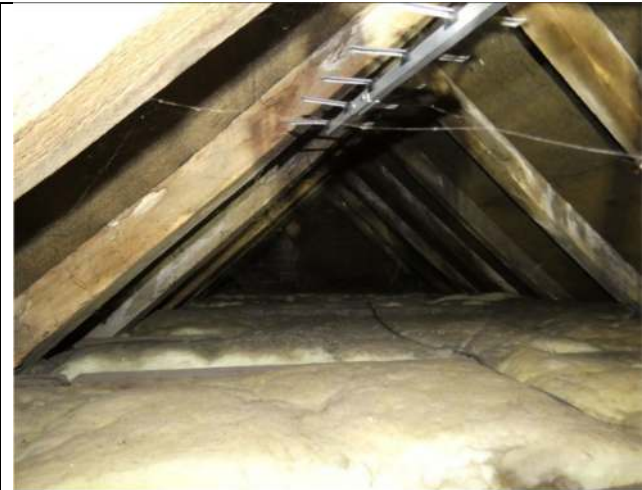
Photograph 43. Part of the enclosed roof void within the main part of The Granary
