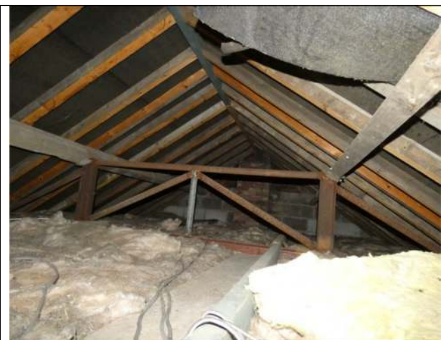
Photograph 41. The enclosed roof void within the single-storey section at the north-east end of The Granary
