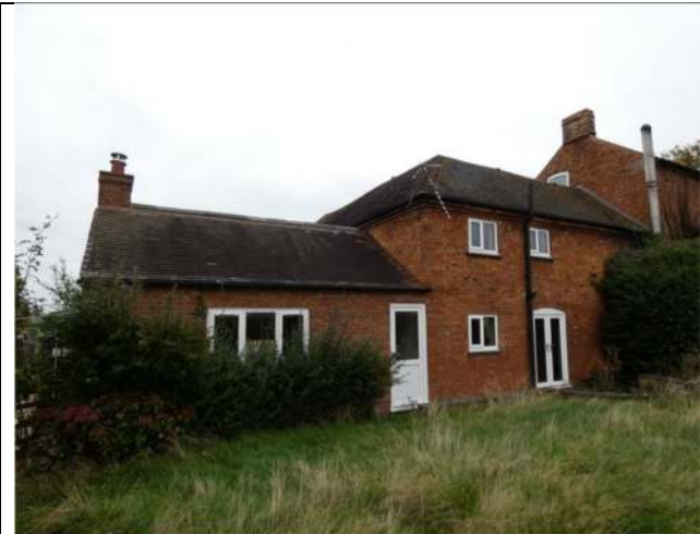
Photograph 31. The north-east elevation of The Granary
