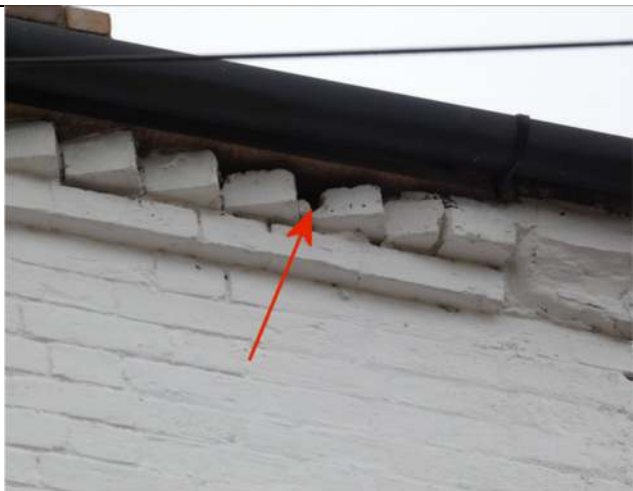
Photograph 17. Opening in the corbelling at the south-east end of the south-west side of the Farmhouse
