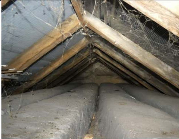
Photograph 19. The section of enclosed roof void in the north-west half of the main part of the Farmhouse (view to north-west)
