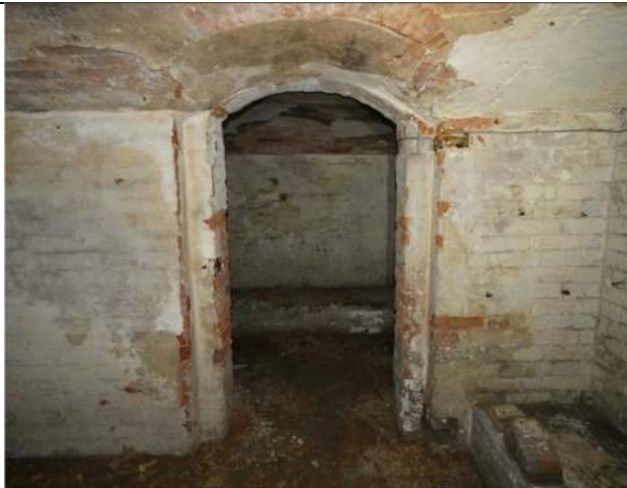
Photograph 27. Example of part of the cellar within the Farmhouse
