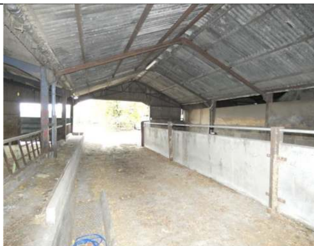
Photograph 58. The interior of Barn 7
