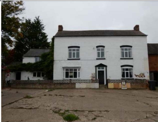
Photograph 1. The south-west elevation of the Farmhouse
