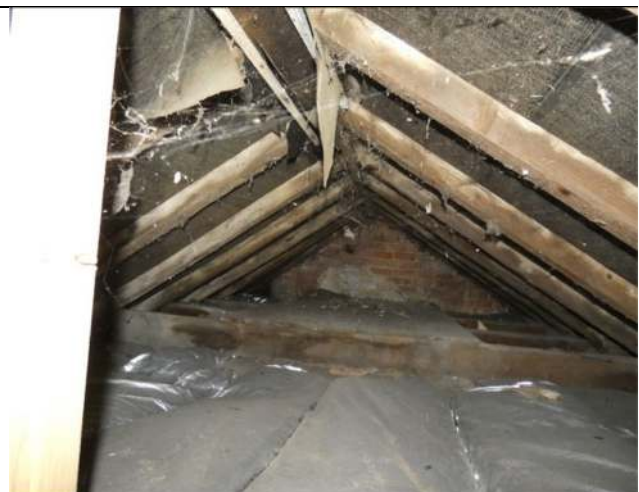
Photograph 24. The section of enclosed roof void within the two-storey section at the north-west end of the Farmhouse
