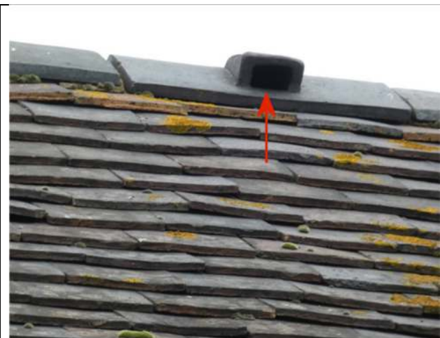
Photograph 33. Example of the ridge vent on the roof of The Granary
