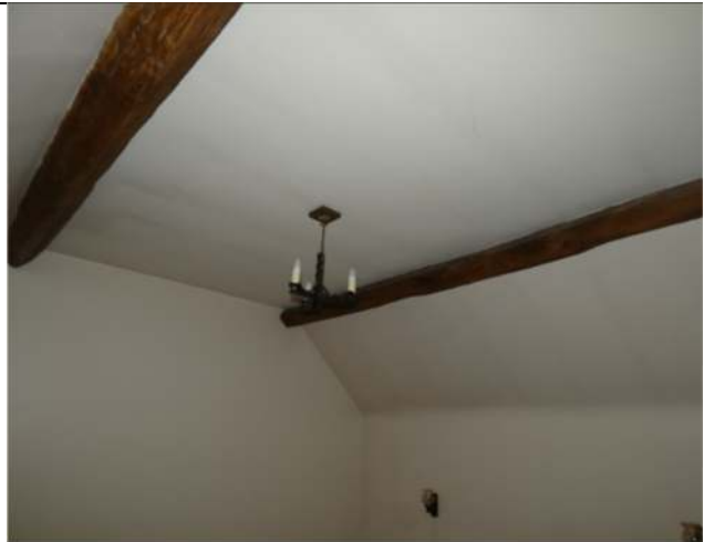
Photograph 44. The part raked ceiling within The Granary
