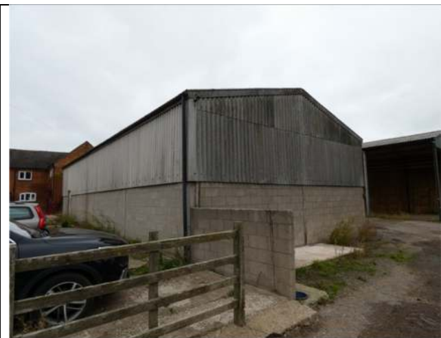
Photograph 45. The north-west and south-west elevations of Barn 3
