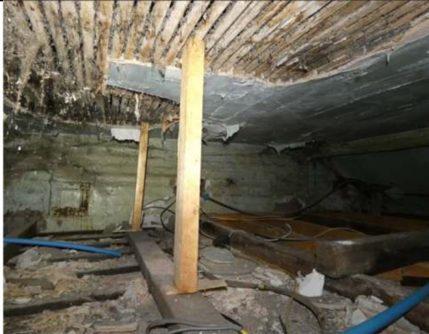
Photograph 25. The section of enclosed roof void within the single-storey section at the north-west end of the Farmhouse (below the laths)
