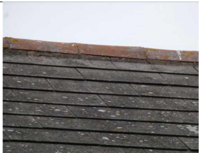
Photograph 6. Example of the slates and tiles on the roof of the main part of the Farmhouse (south-west facing roof pitch)
