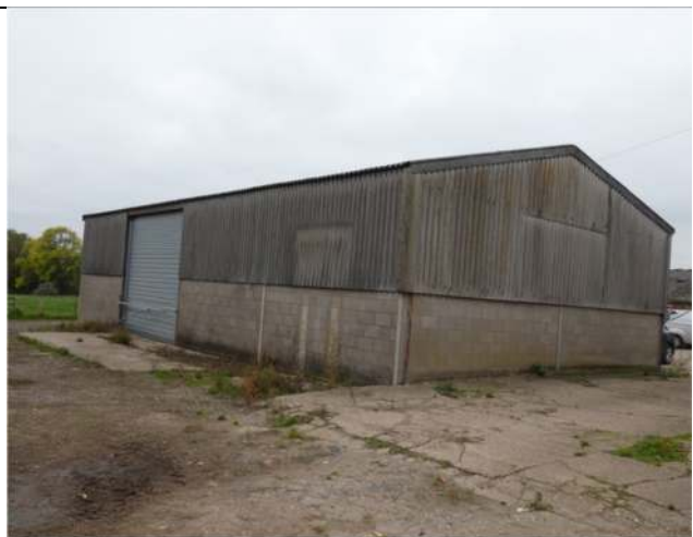
Photograph 46. The north-east and south-east elevations of Barn 3
