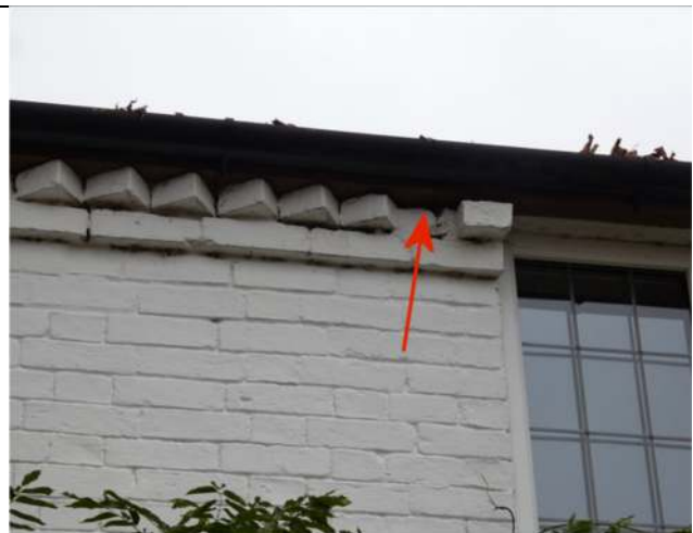
Photograph 18. Opening in the corbelling on the two-section at the north-west end of the Farmhouse
