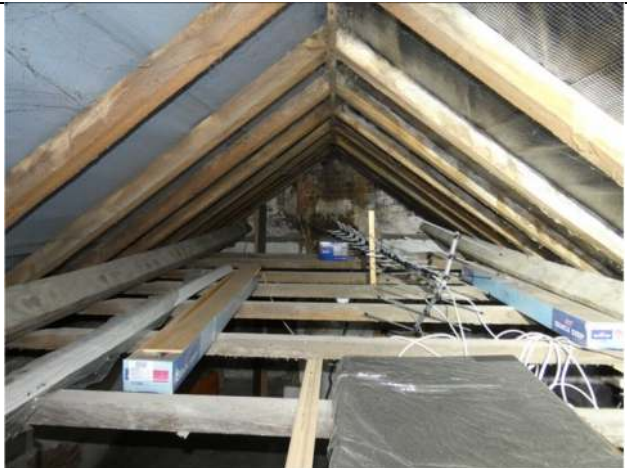
Photograph 21. The roof void in the south-east half of the main part of the Farmhouse (view to south-east)
