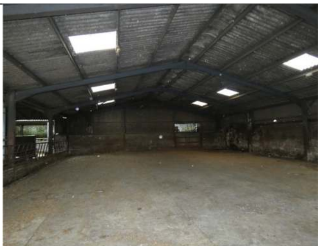
Photograph 57. The interior of Barn 6
