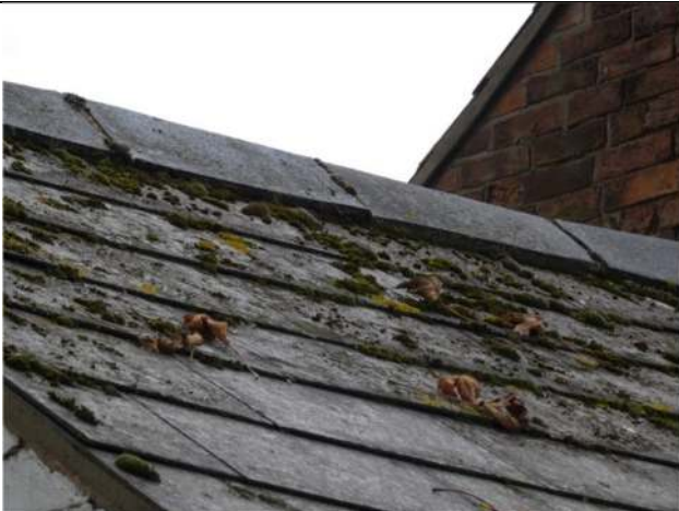
Photograph 9. Example of the slates on the 2 section at the north-west end of the Farmhouse
