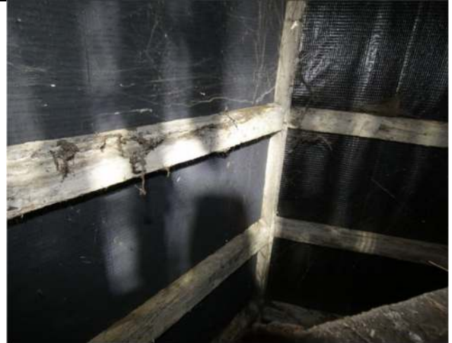
Photograph 26. The section of enclosed roof void within the single-storey section at the north-west end of the Farmhouse (above the laths)
