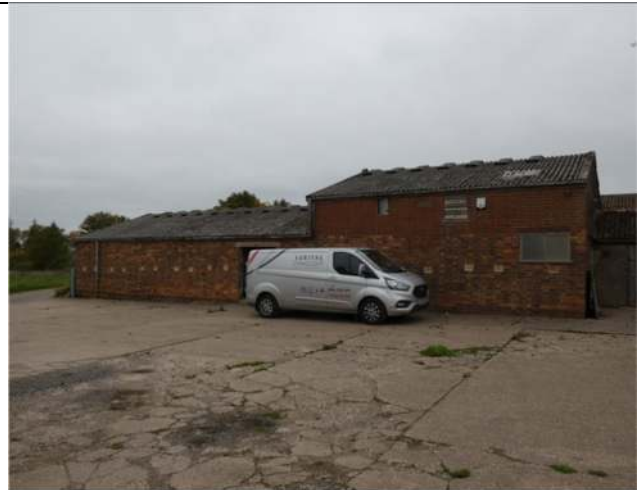
Photograph 50. The south-east elevation of Barn 5
