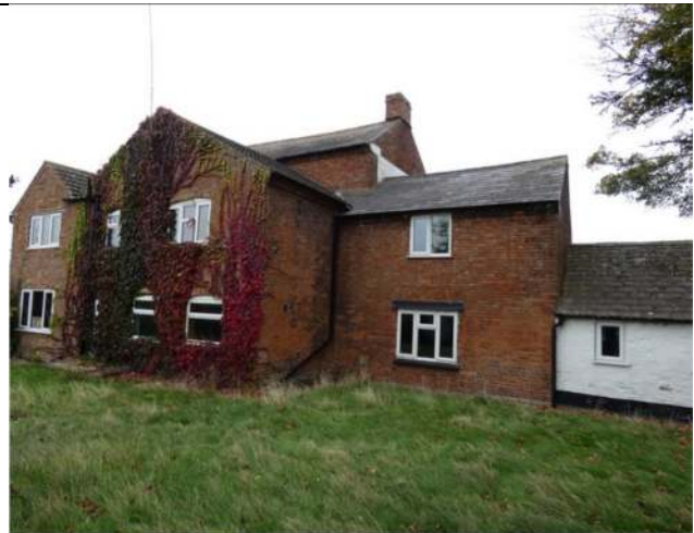
Photograph 4. The north-east elevation of the Farmhouse
