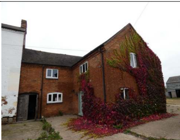
Photograph 29. The south-west and north-west elevations of The Granary
