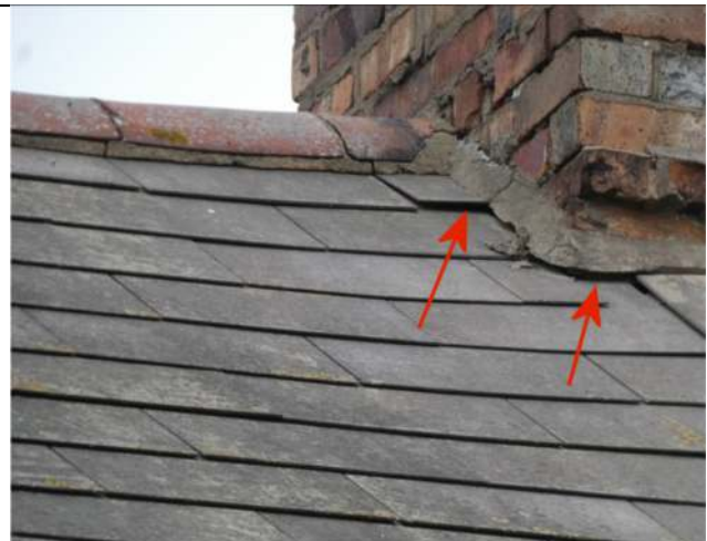
Photograph 12. Example of the sealed lead flashing at the base of the chimney on the Farmhouse
