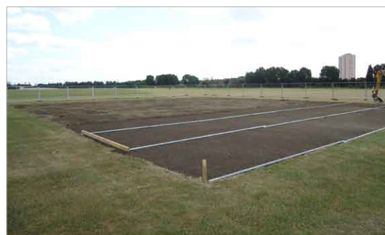
Precise placement and consolidation of cricket loam is crucial to the success of cricket square construction
