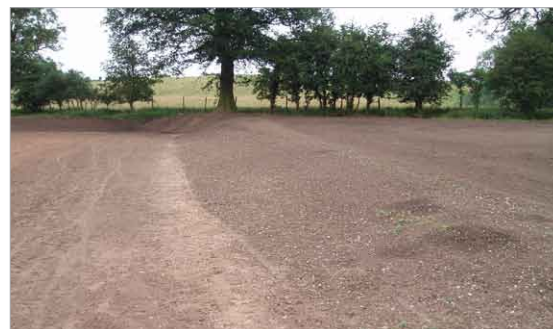
Slopes of surrounding banks should not exceed 1 in 3 to facilitate mowing
