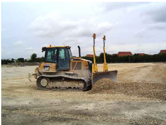
Laser-guided grading of a pitch
