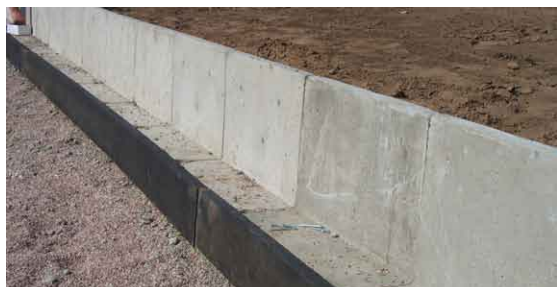
Pre-formed ditch channel simplifies construction
