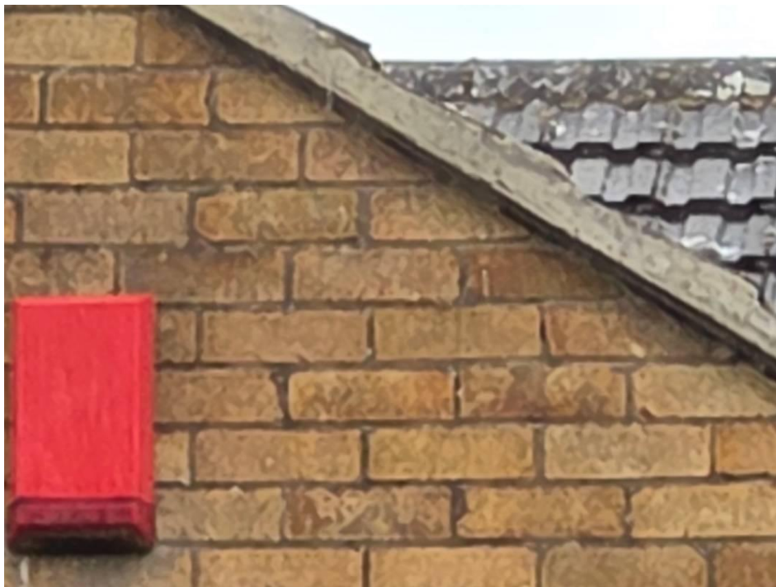
Photograph 7: Feature 1 of the main building.
