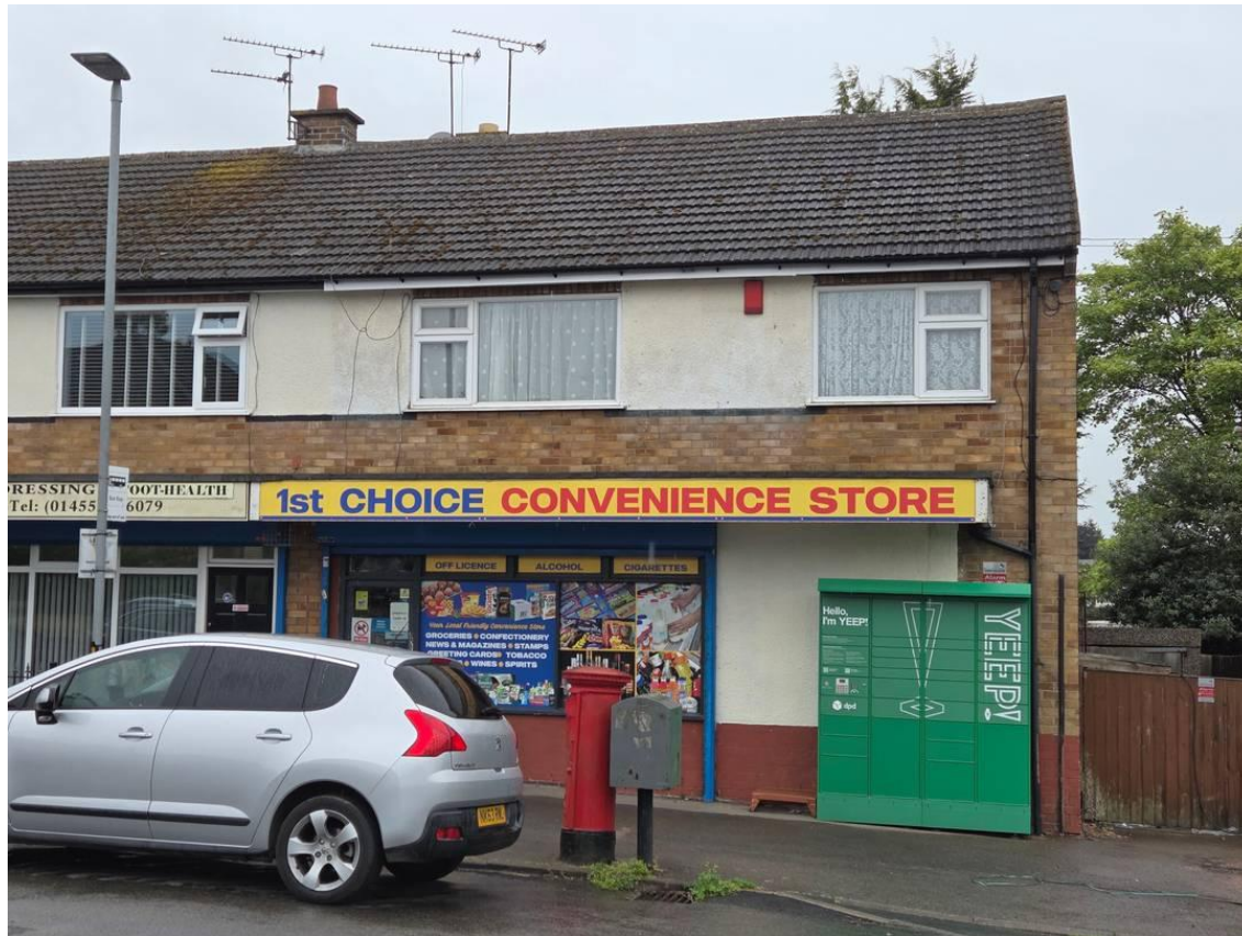
Photograph 1: The northern elevation of the main building.
