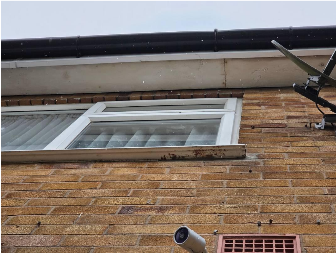
Photograph 9: Feature 3 of the main building.
