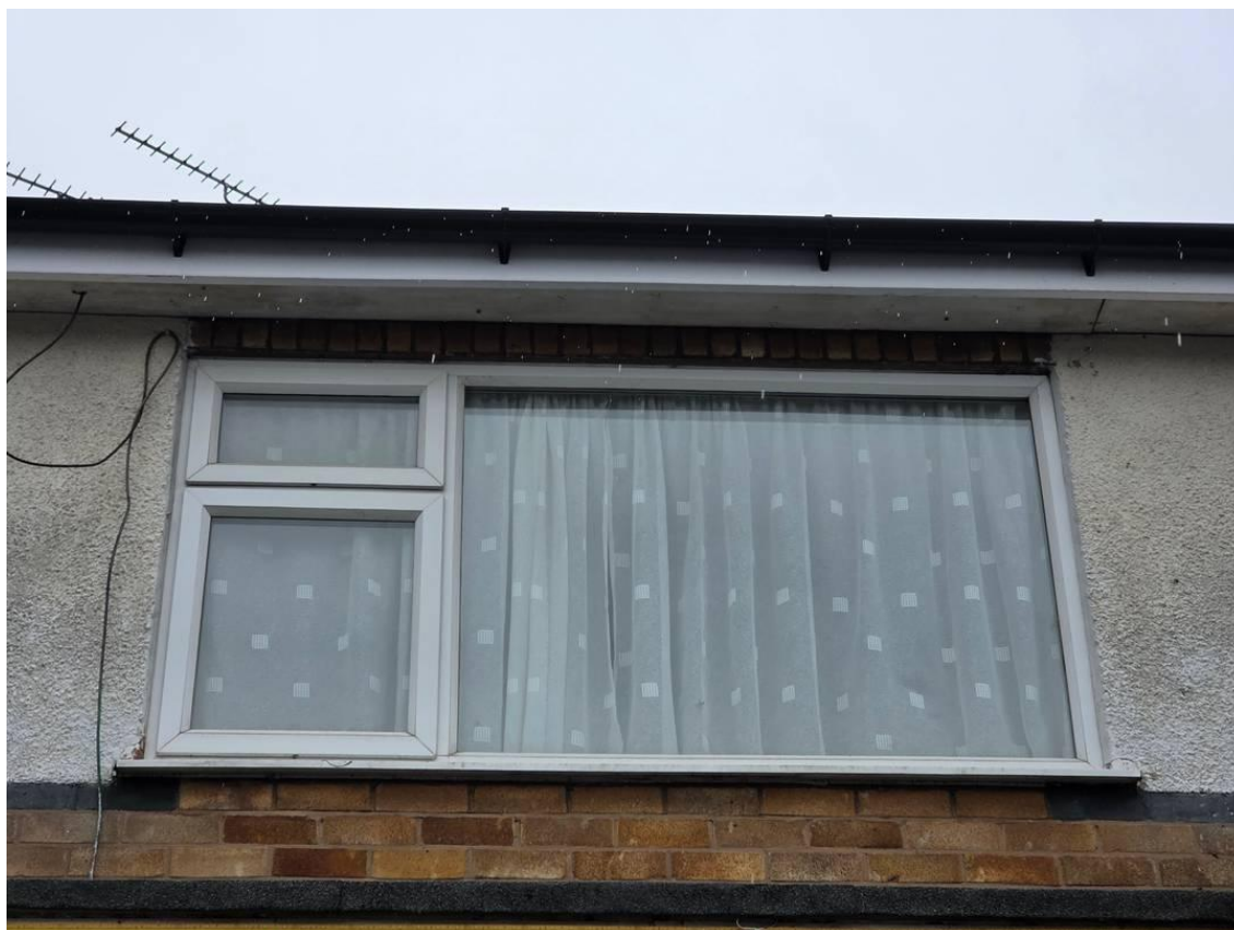
Photograph 8: Feature 2 of the main building.
