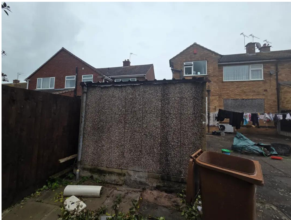
Photograph 5: The southern elevation of Building 2.
