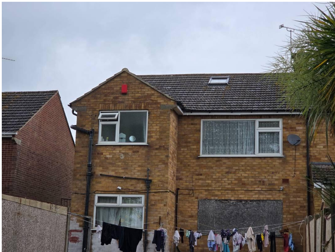
Photograph 2: The southern elevation of the main building.
