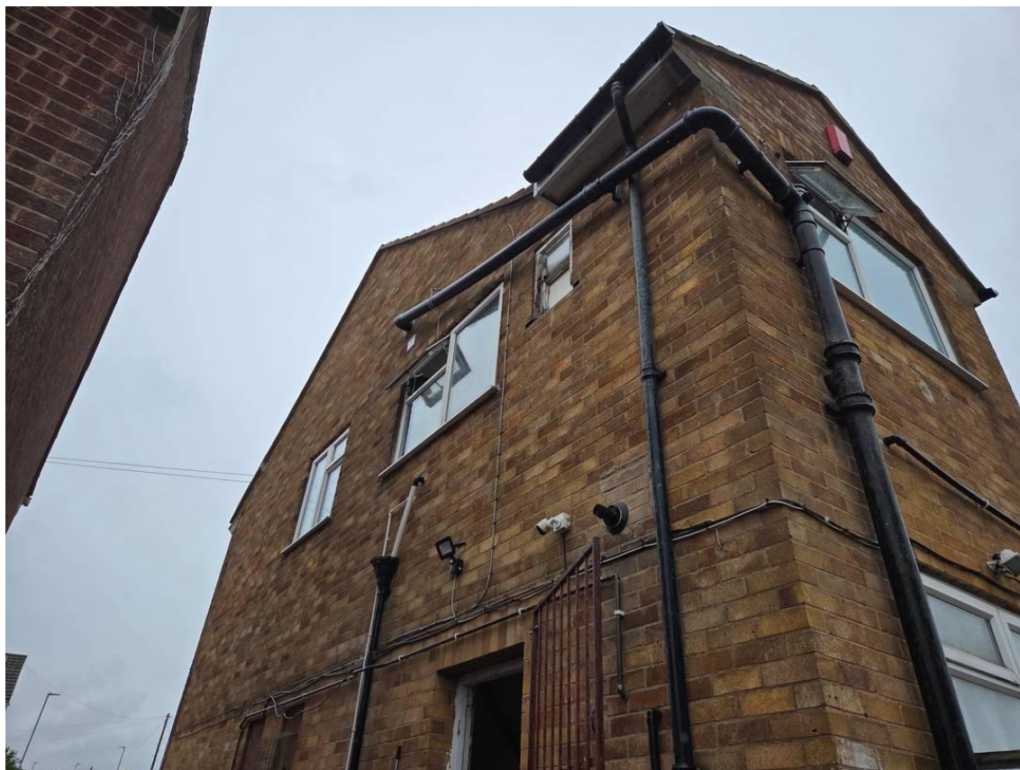
Photograph 3: The eastern elevation of the main building.
