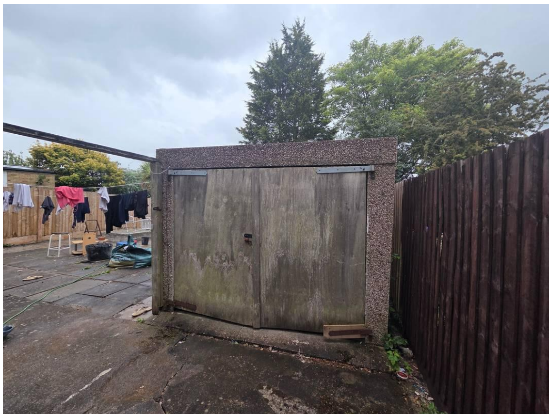
Photograph 4: The northern elevation of Building 2.
