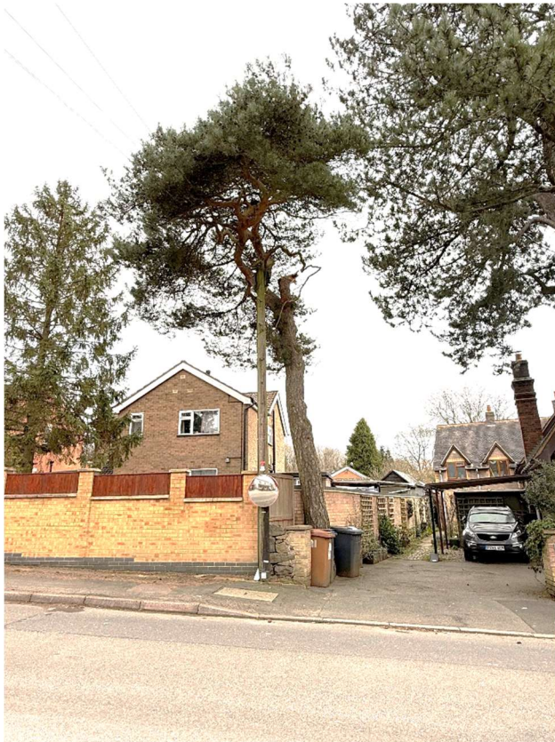
Photograph 5: Showing the heavily offset crown of tree 1 over the neighbouring property, post storm damage.
