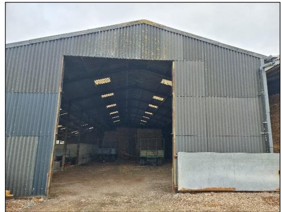
Figure 3: Eastern elevation of Building 5 showing interior of floorspace subject of change of use to Class B8.
