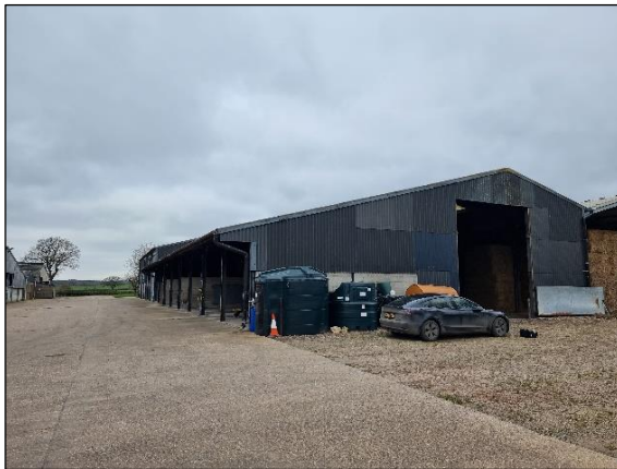
Figure 2: Facing west towards Building 5, showing open-sided lean-to to be retained in agricultural use
