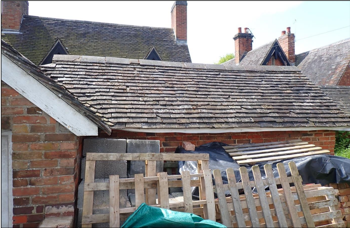
Photograph 5: Rear view of the attached brick-built outbuilding taken from the north
