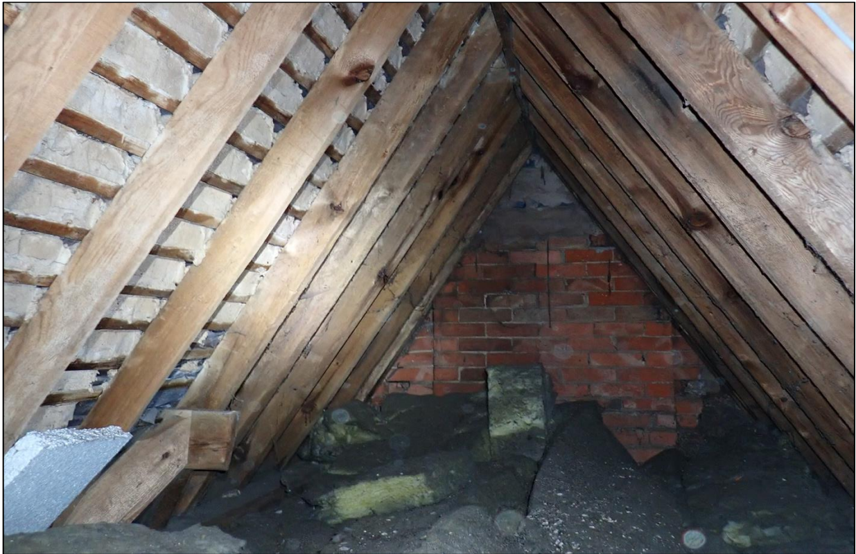
Photograph 3: Internal view of the main two-storey dwelling showing the open couple roof structure with mortar torching and fibre-glass insulation covering the floor
