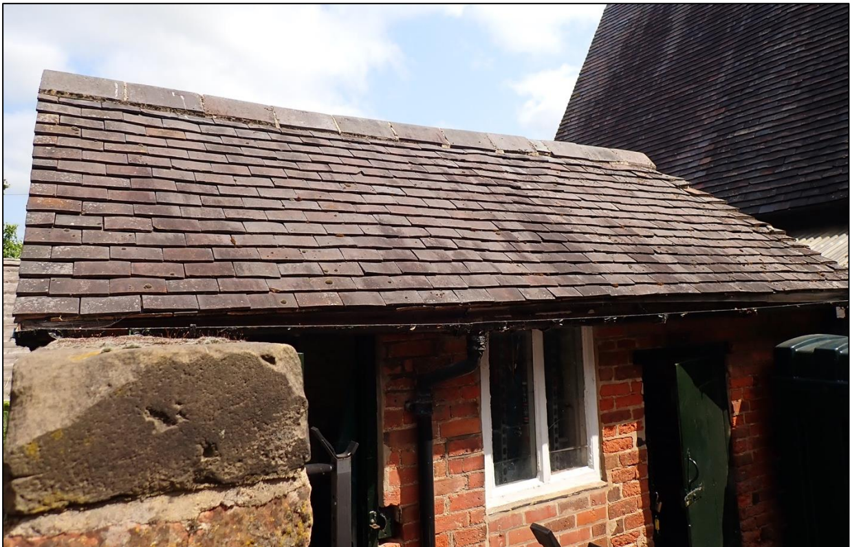
Photograph 4: Front view of the attached brick-built outbuilding taken from the south
