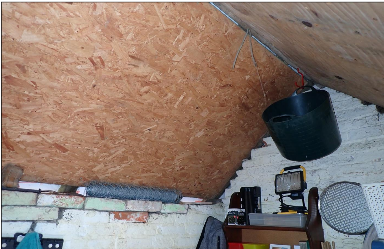
Photograph 6: Internal view of the attached brick-built outbuilding showing the vaulted chipboard ceiling
