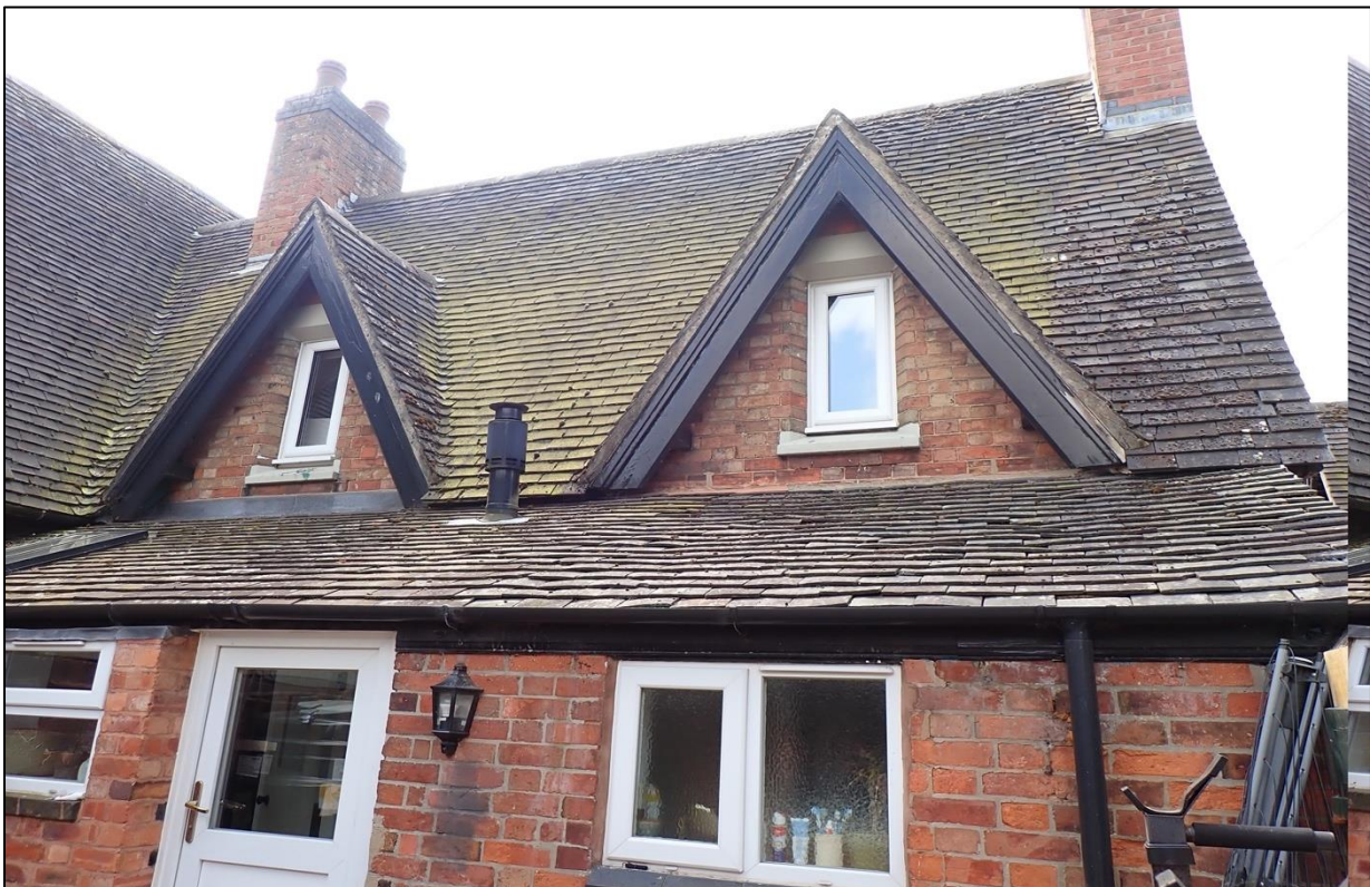
Photograph 2: Rear view of the main two-storey dwelling taken from the north, showing the uPVC windows and doors
