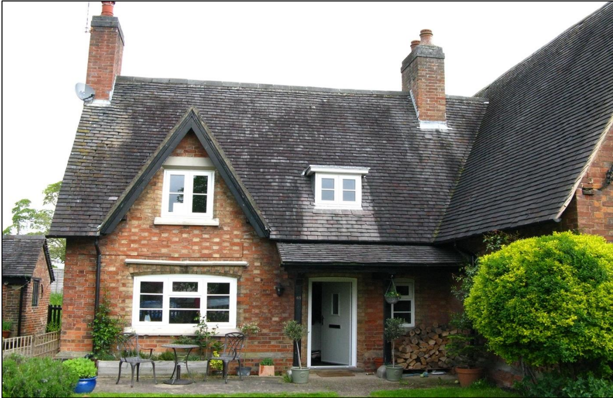
Photograph 1: Front view of the main two-storey dwelling taken from the south showing the plain clay tiled roof
