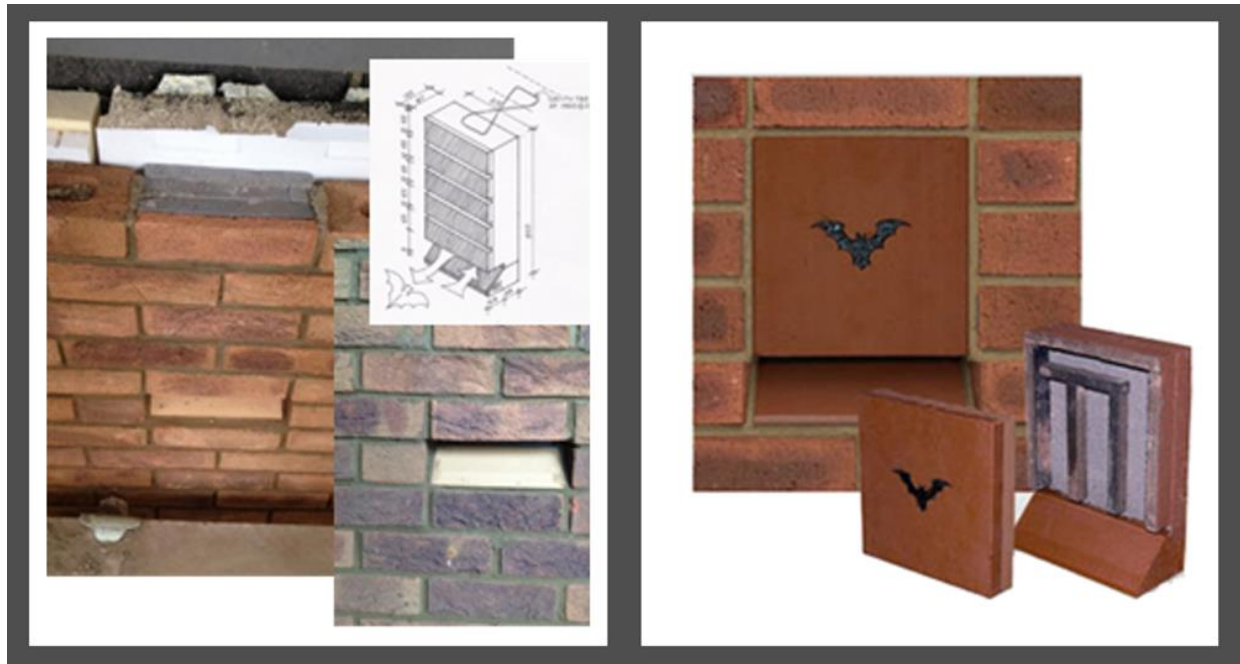
Figure 4 - example of the integrated bat boxes
