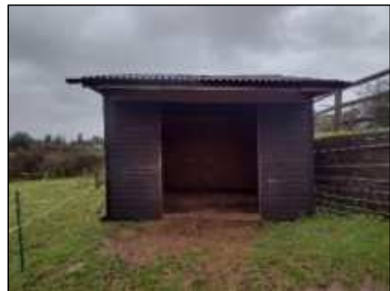
Photograph 25: Field Shelter 'B4'
