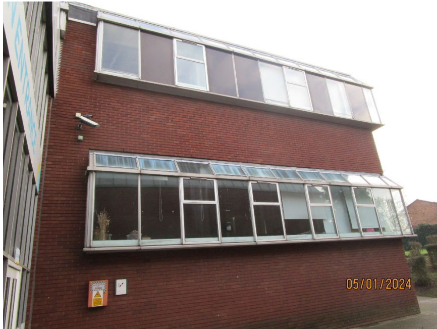
West facing elevation showing windows for replacement.
