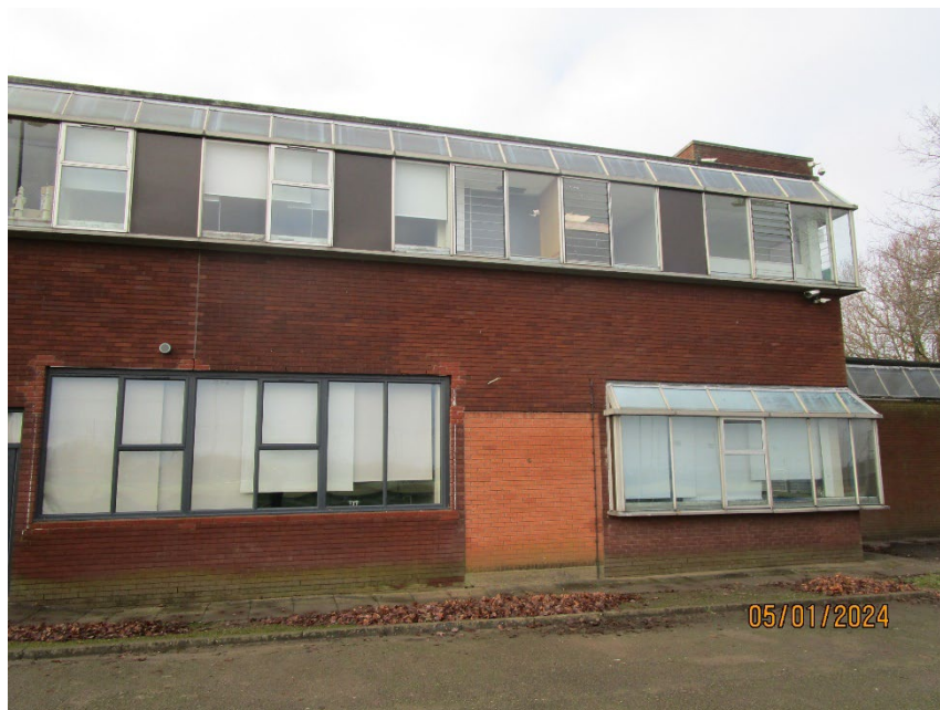
East facing elevation showing windows for replacement.
