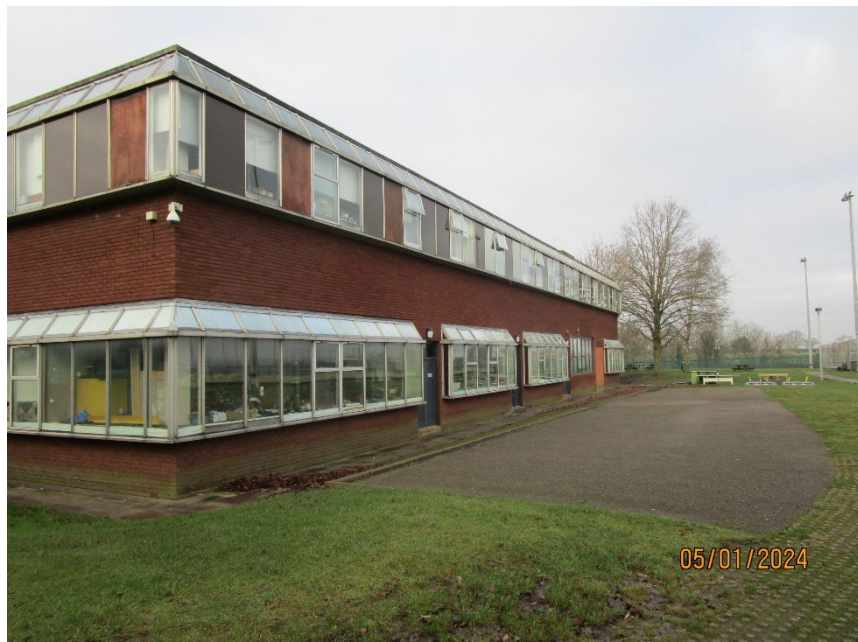
East facing elevation showing windows for replacement.
