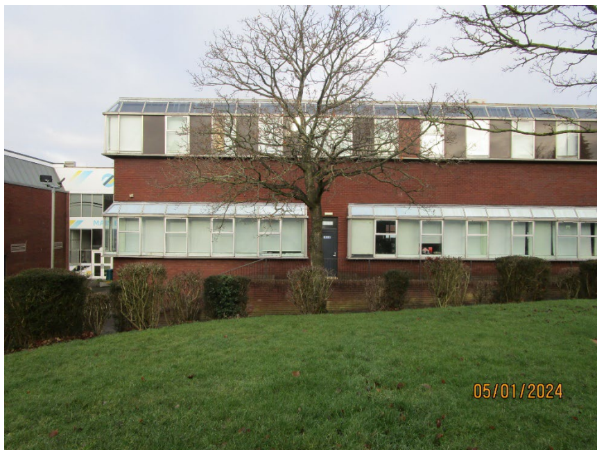
South facing elevation showing windows for replacement.
