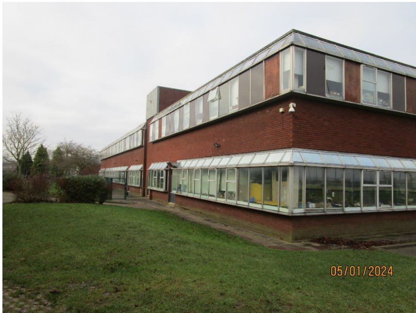
South facing elevation and corner of East elevation showing windows for replacement.
