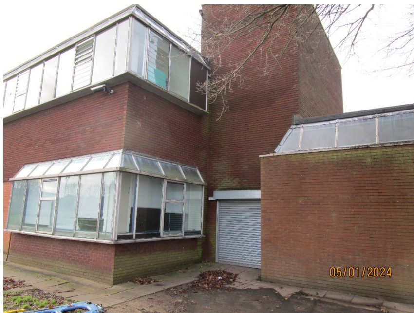
North facing elevation showing windows for replacement.
