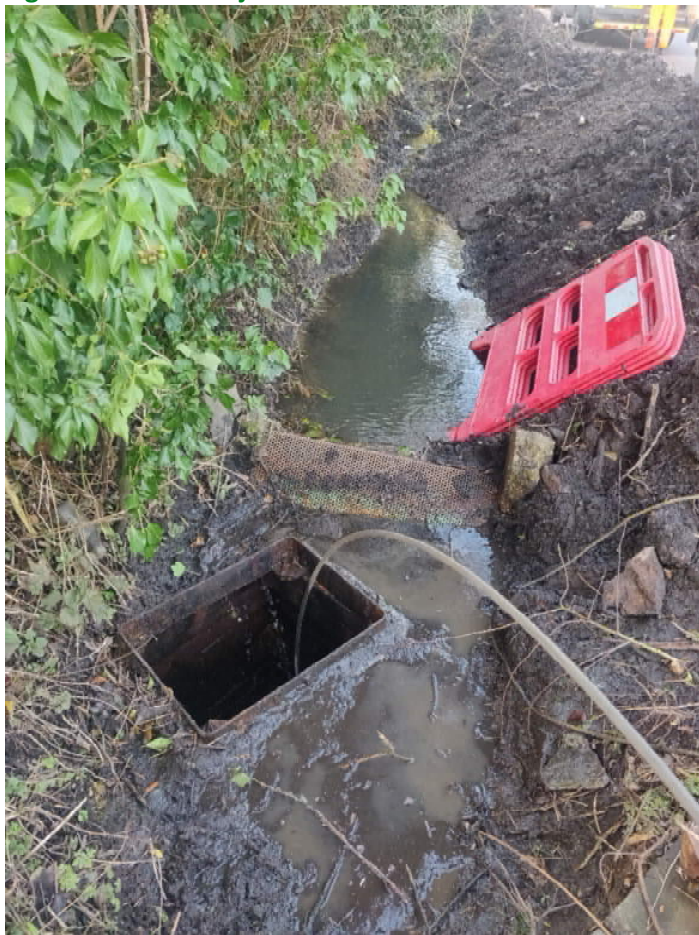
Figure 4.1: Ditch adjacent to site
