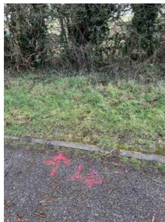
11_MH01_Downstream_DS.jpg, 00:10:30, 58.99 m General photograph taken at this point, Position traced & marked 1.4m deep
