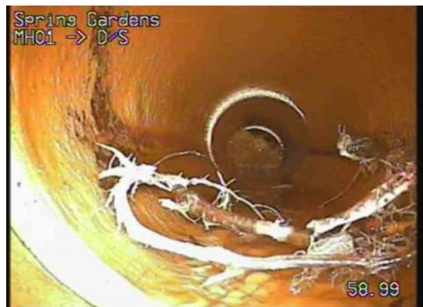
9_MH01_Downstream_DS.jpg, 00:10:29, 58.99 m Survey abandoned, Unable to pass tap roots
