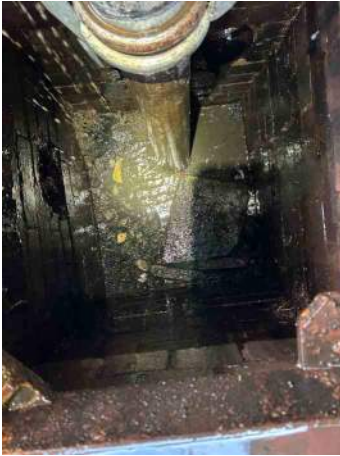
2_MH01_Downstream_DS.jpg, 00:00:00, 0.00 m Start node, catchpit, reference: MH01
