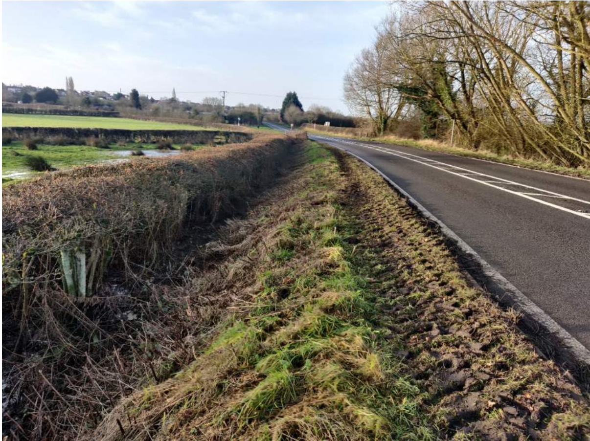
Ditch adjacent to Leicester Road road looking west towards unnamed road
