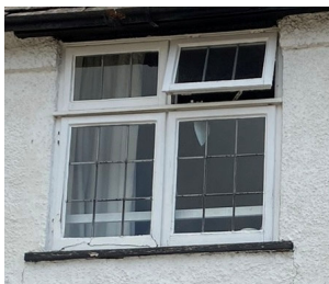
Existing Window Image
