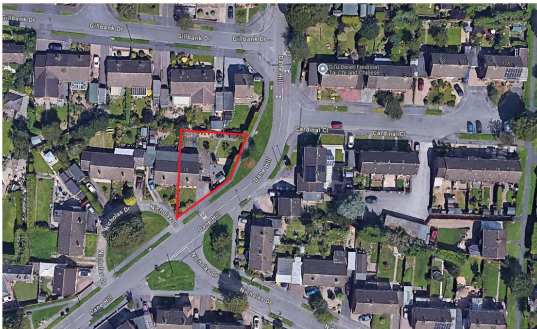
Approximate extent and location of the Site
