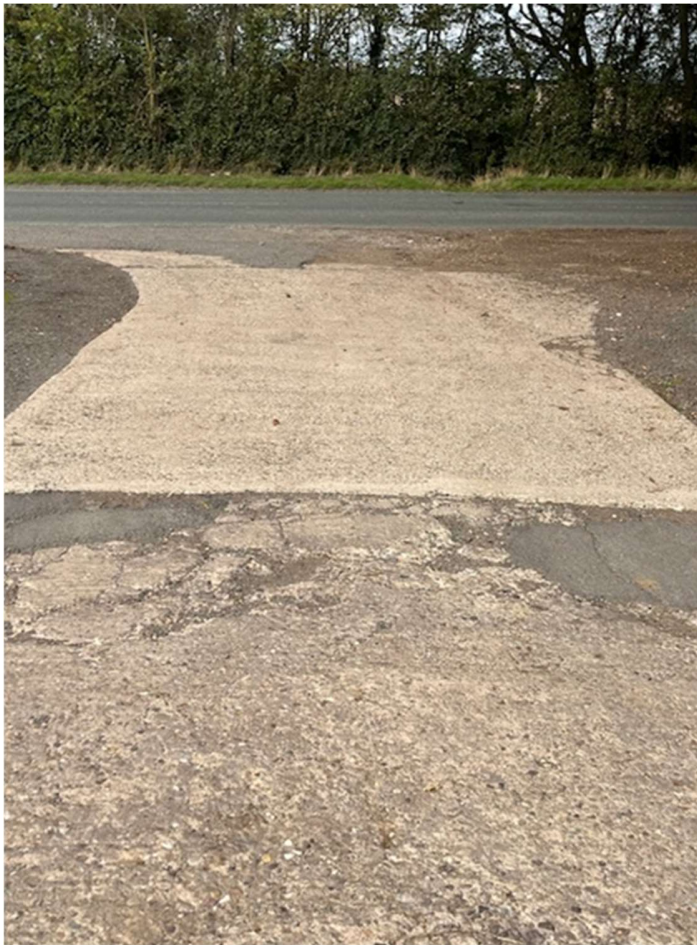
Figure 5 Concrete sealed surface at the end of the access road leading to Fenn lanes
