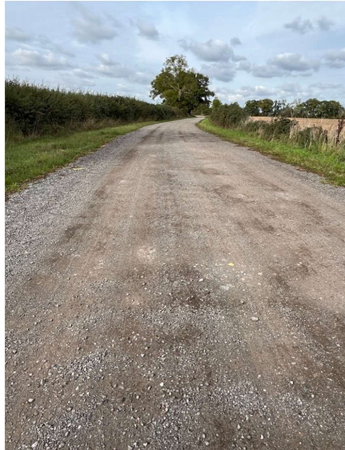
Figure 4 Unsealed access road leading to Fenn Lanes
