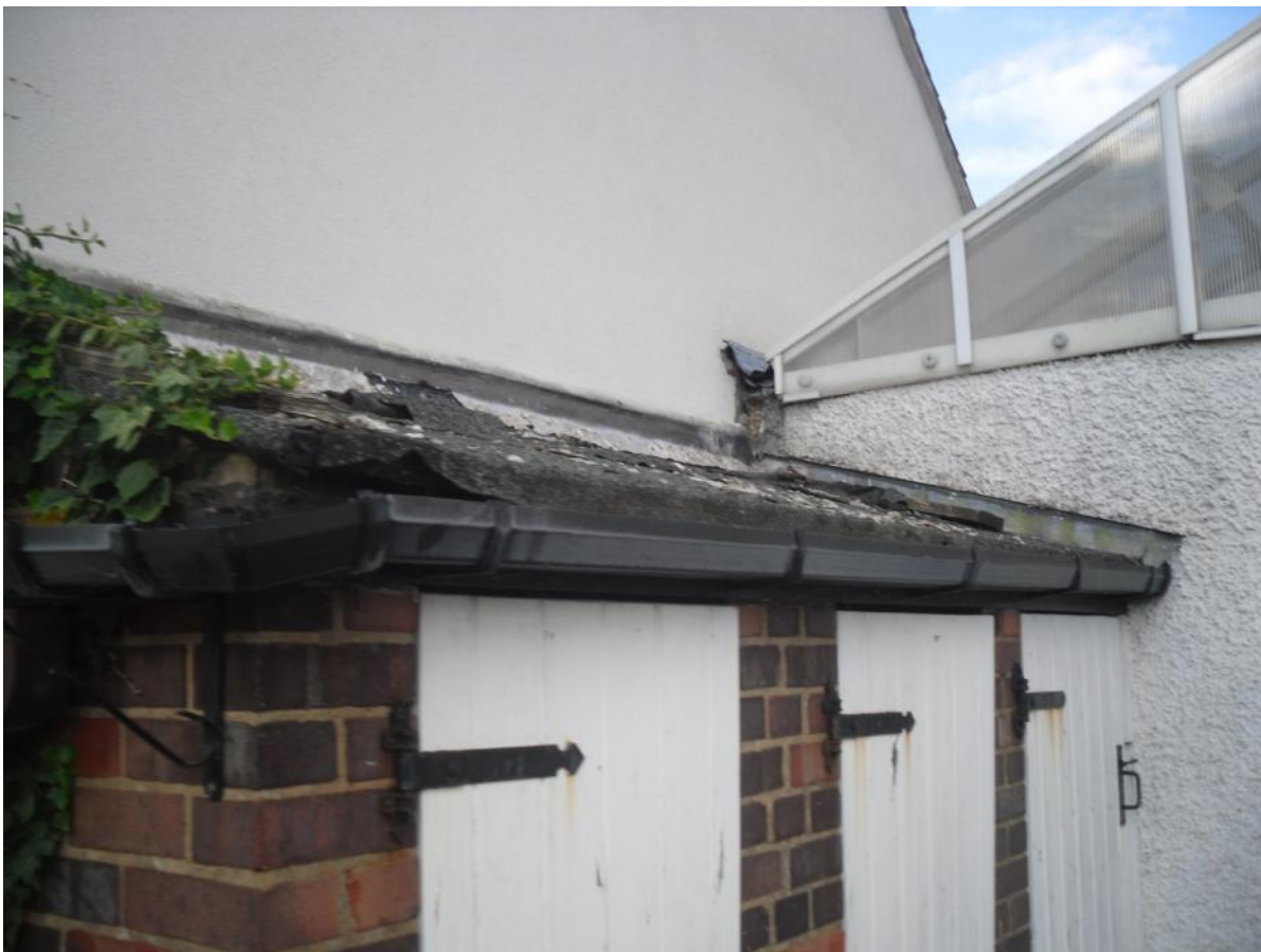
Single storey outside toilets/sheds: no cavity, mineral roof intact
