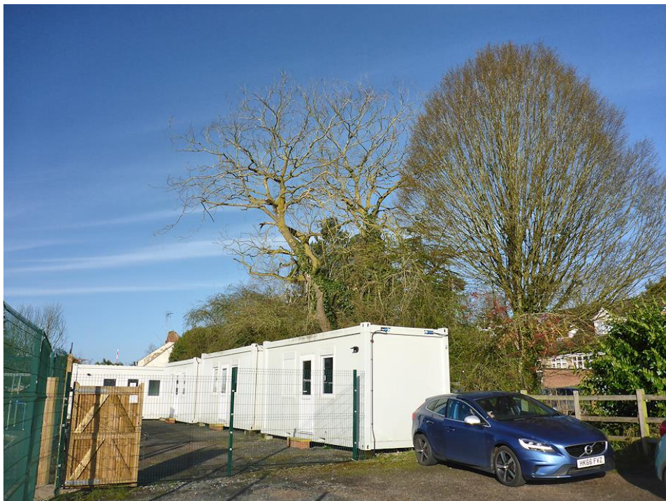
The current temporary classrooms looking northwest.
