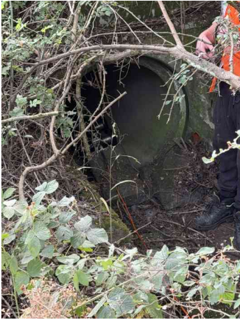
Culvert Header Wall
