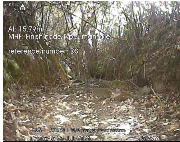
2, 00:02:00, 15.79 m Finish node, manhole, reference: DS
