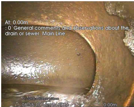
1, 00:00:03, 0.00 m 0`General comments and observations about the drain or sewer., Main Line
