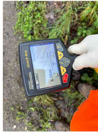
MAIN LINE INVERT 0.98M
