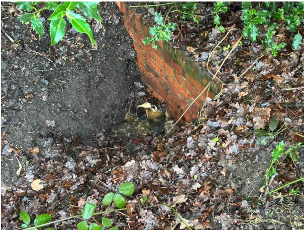
HEADWALL INVERT 840MM TO TOP OF BRICKS
