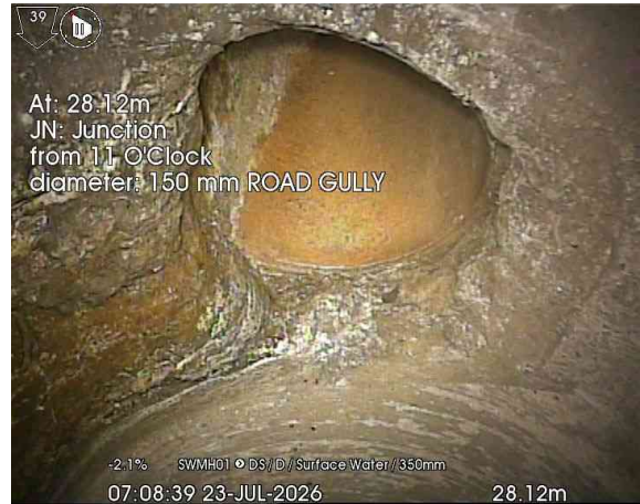
6, 00:03:57, 28.12 m Junction at 11 o'clock, 150mm dia, ROAD GULLY
