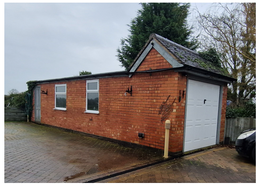
View of garage from the house
