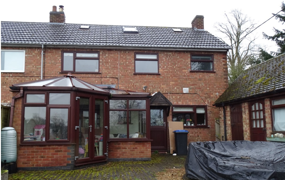
Image 3 – Rear West facing elevation of the property
