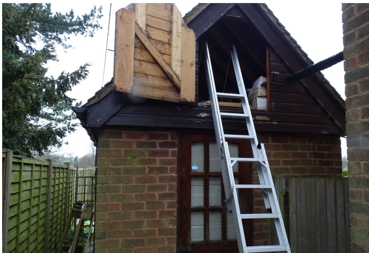
Image 8 – East facing elevation of the detached outbuilding as above
