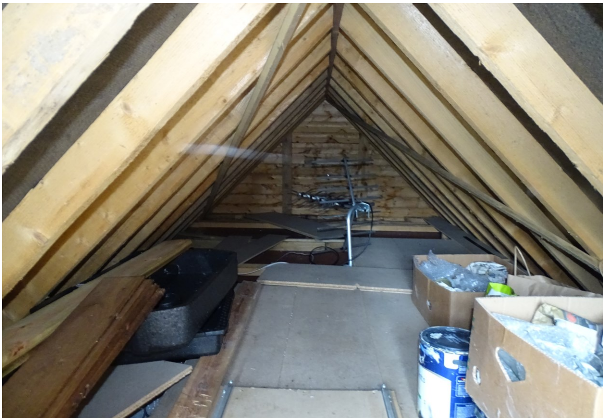
Image 10 – Internal view from within the roof void spaces of the detached outbuilding
