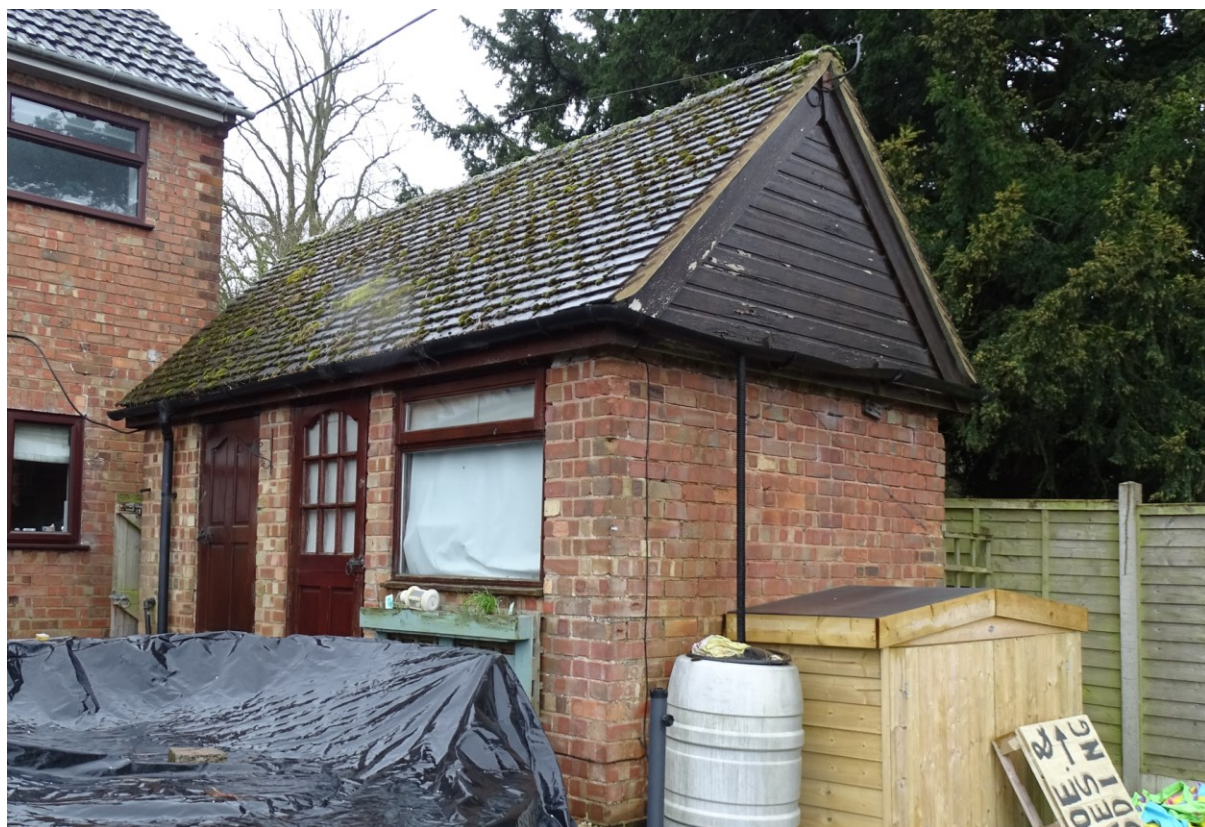
Image 7 – North & West facing elevation of the rear outbuilding structure
