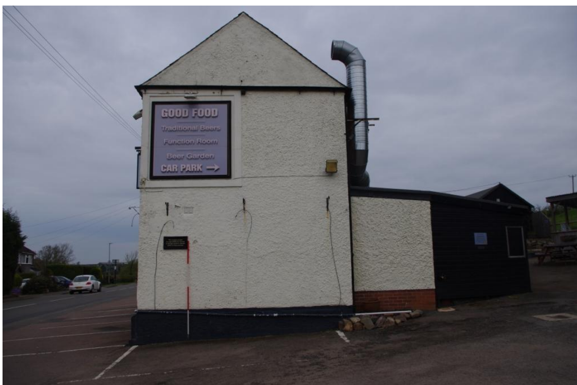
Figure 11 Building A , East – South East Facing Elevation (Looking West – North West).
