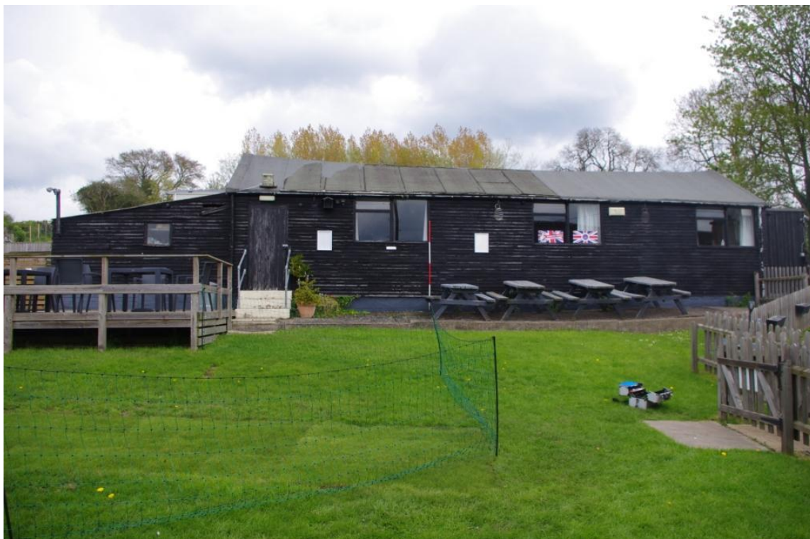
Figure 22 Building B , South – South East Facing Elevation (Looking North – North East).
