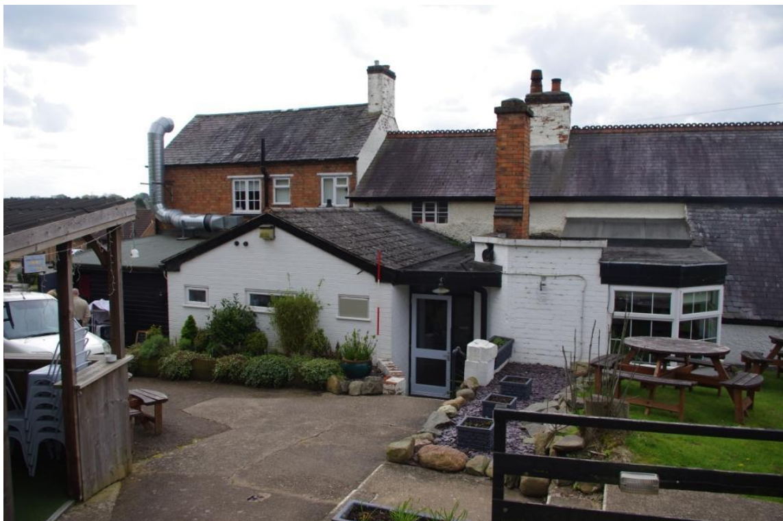
Figure 14 Building A , Rear Elevation (Looking South).
