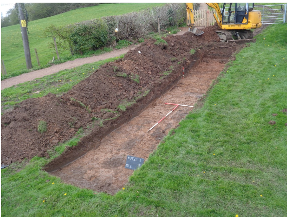
Plate 8; trench 2, view northwest.
