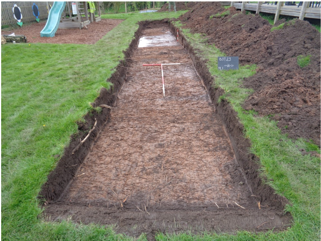
Plate 2; trench 1 view west.
