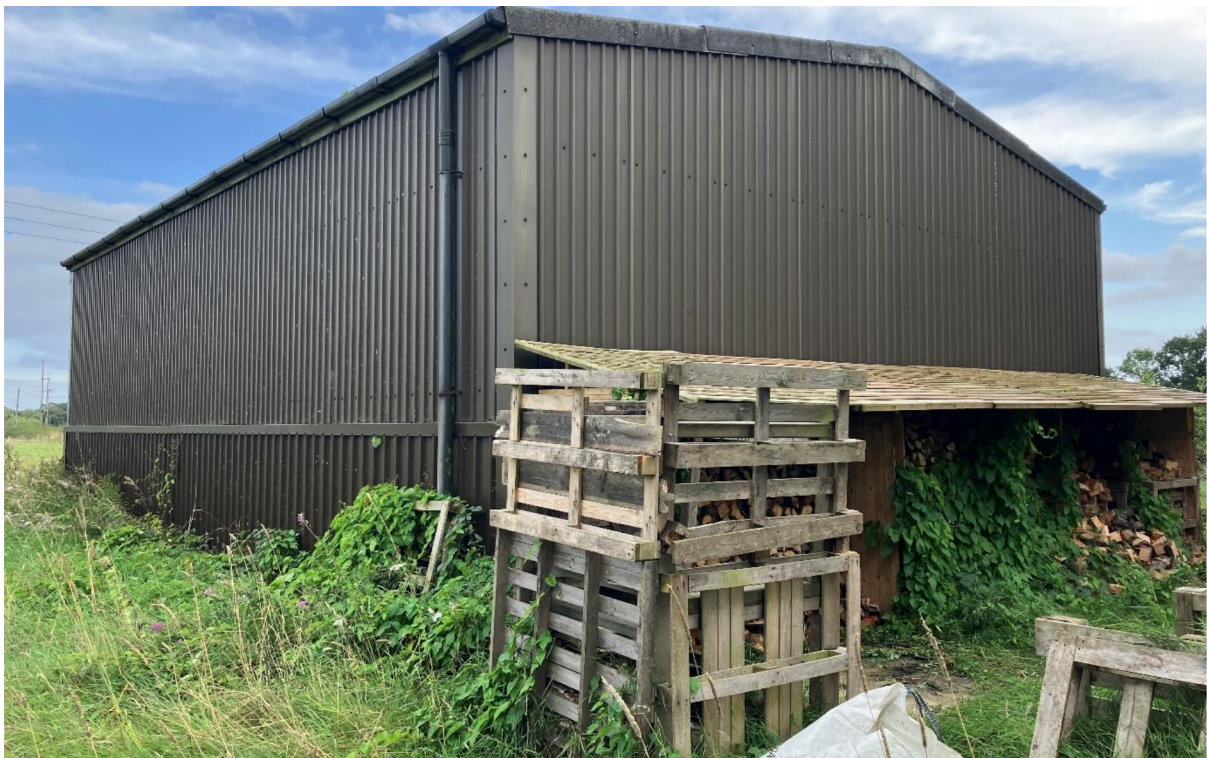
Existing Building – External photo
