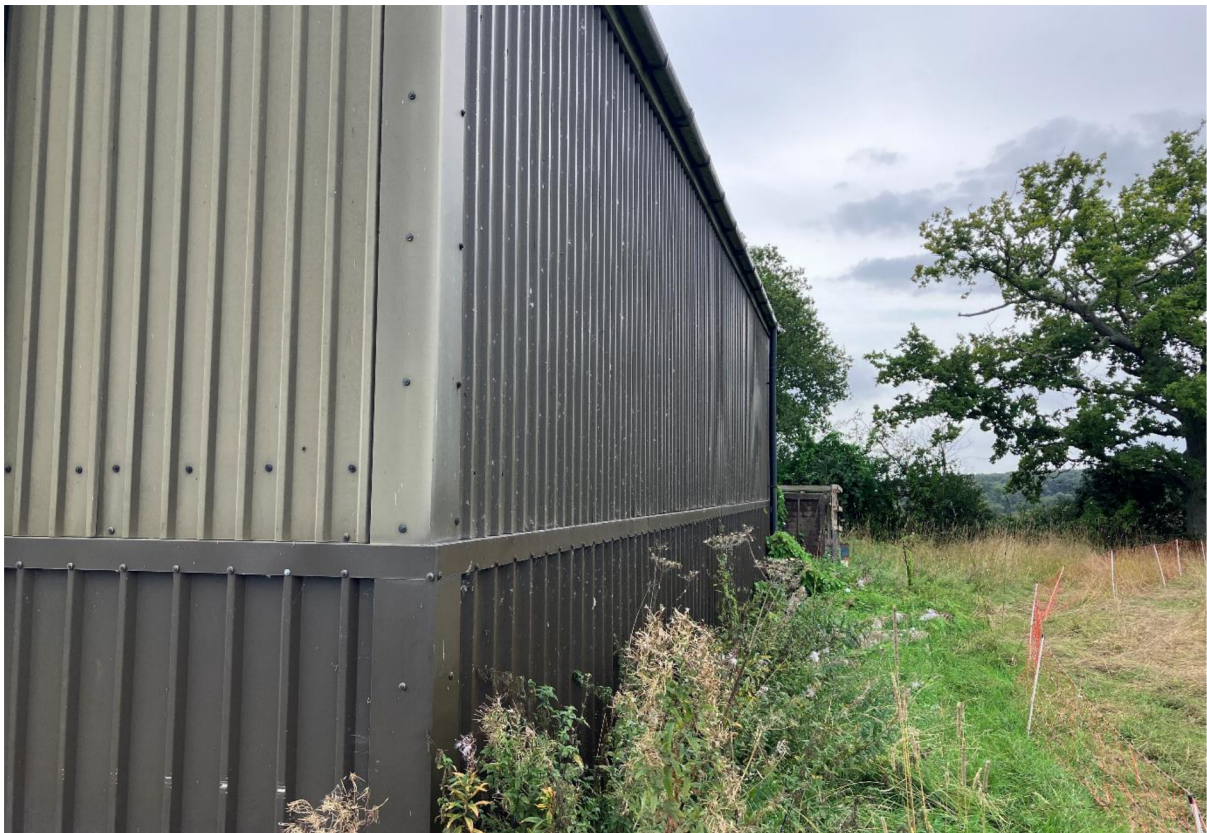
Existing Building – External photo
