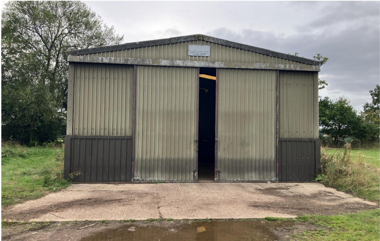
Existing Building – External photo
