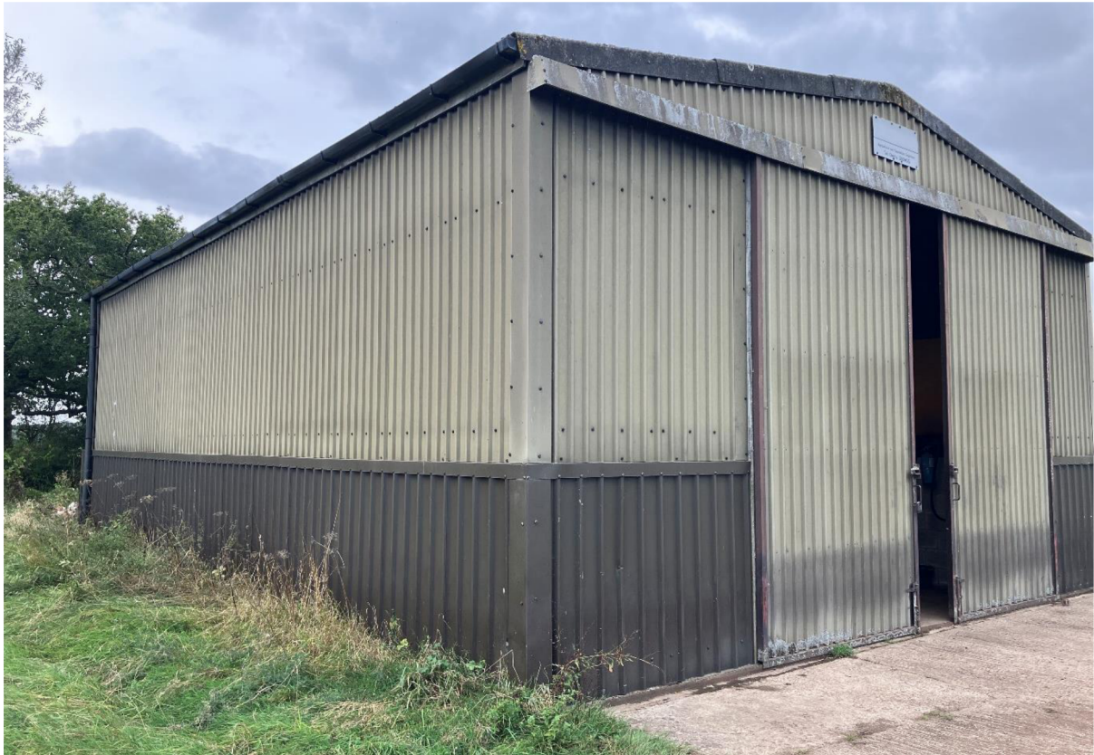
Existing Building – External photo
