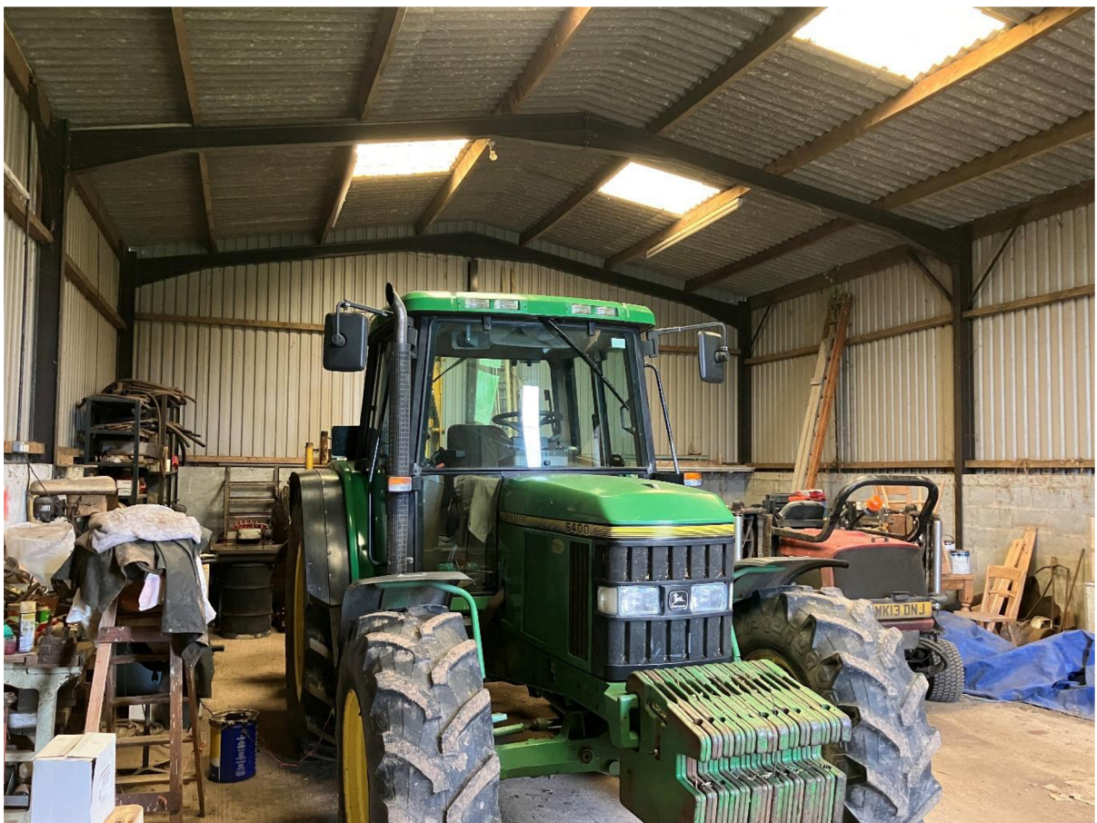
Existing building – internal image
