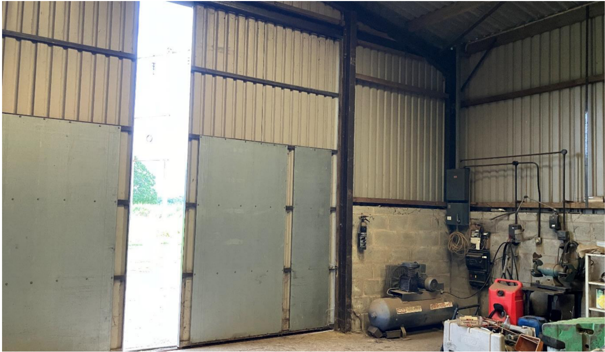
Existing building – internal image
