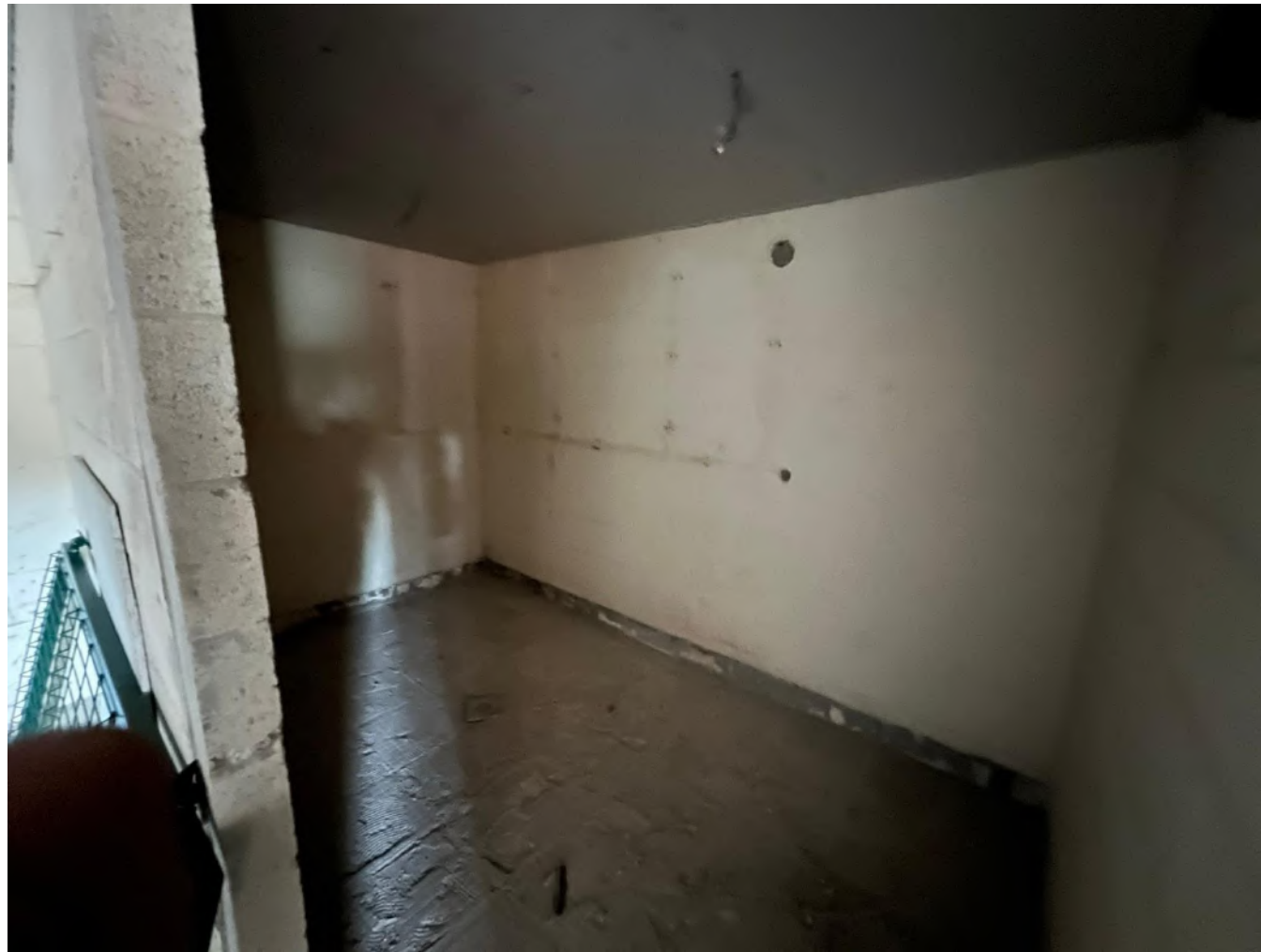
Shower area: Before
