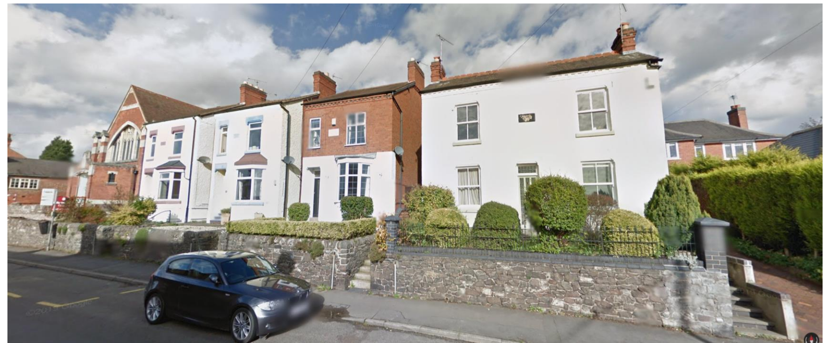
Houses along Station Road feature both red brick and white render.
