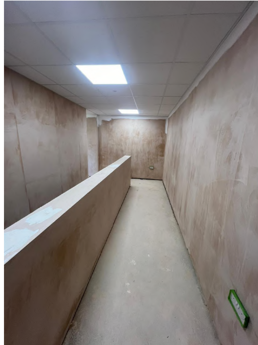
First floor landing
