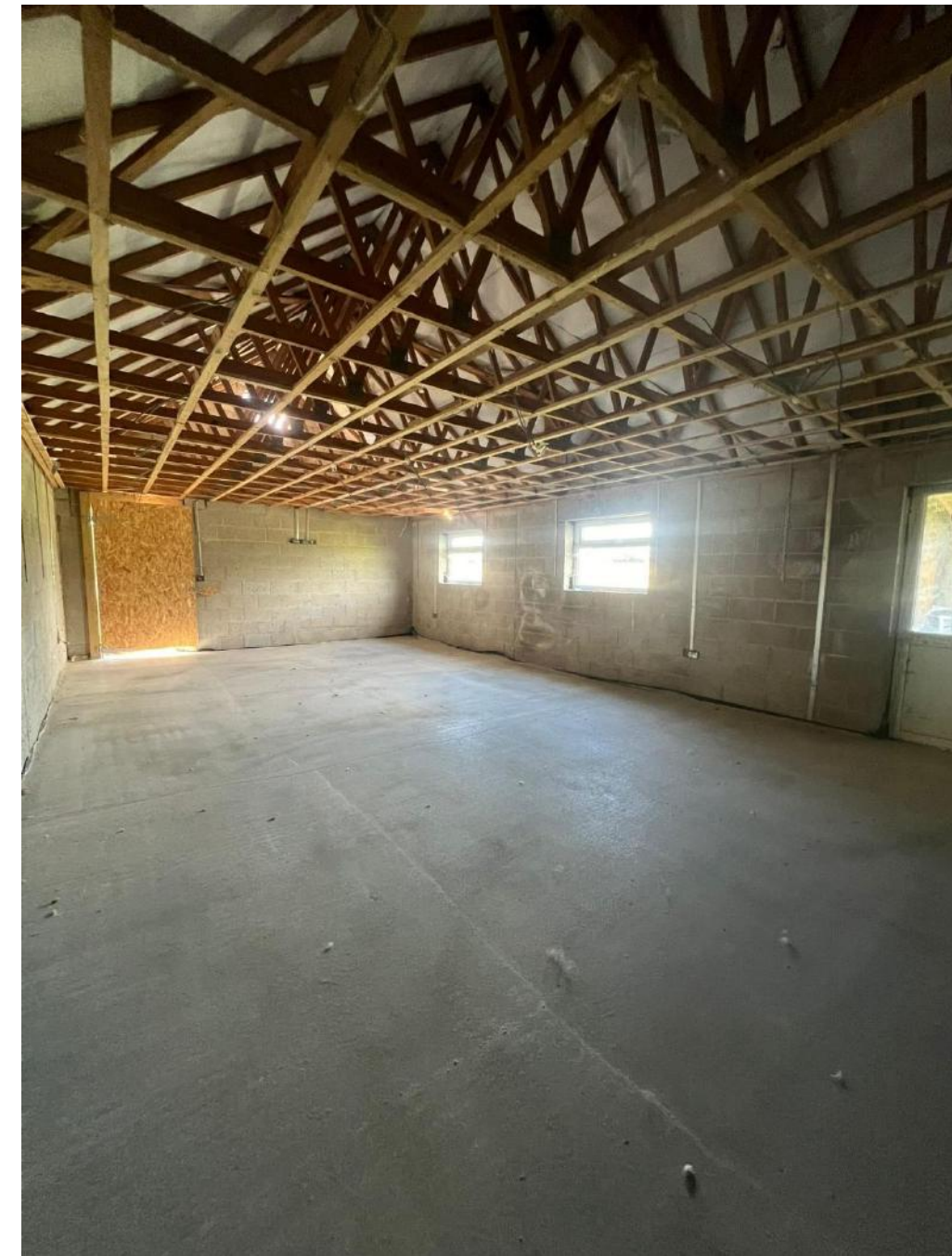
First floor club room: After (still to be completed)
