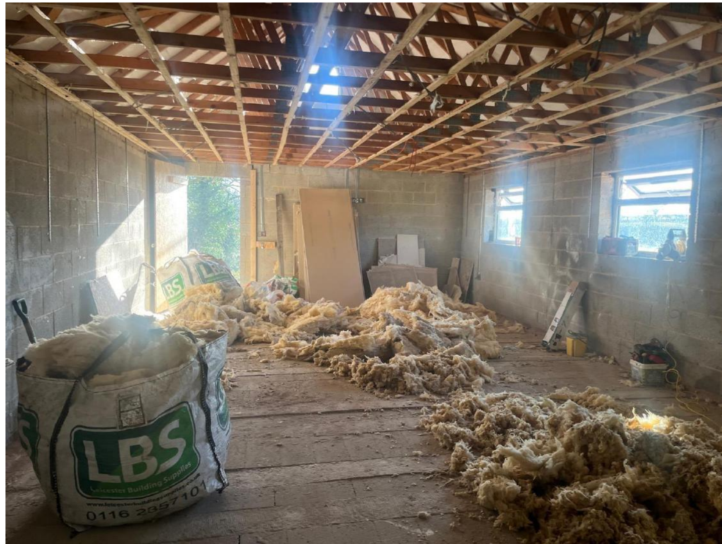
First floor club room: Before
