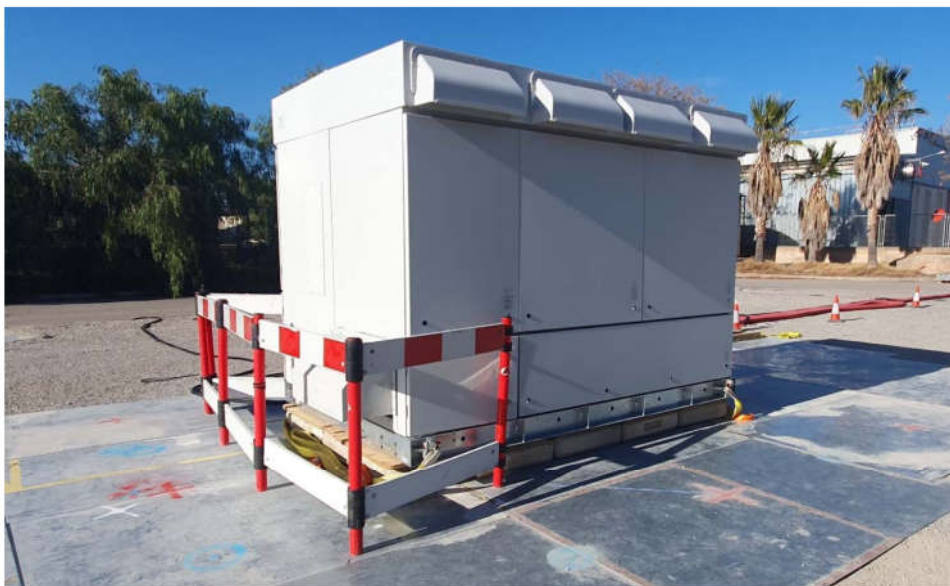
Illustration 6. Views of the PCSK Gen3 inverter without acoustic attenuation kit
