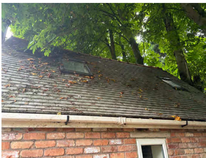
Image 3 - Northern elevation of B1, and general condition of roof tiles.
