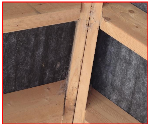
Internal view of barn
