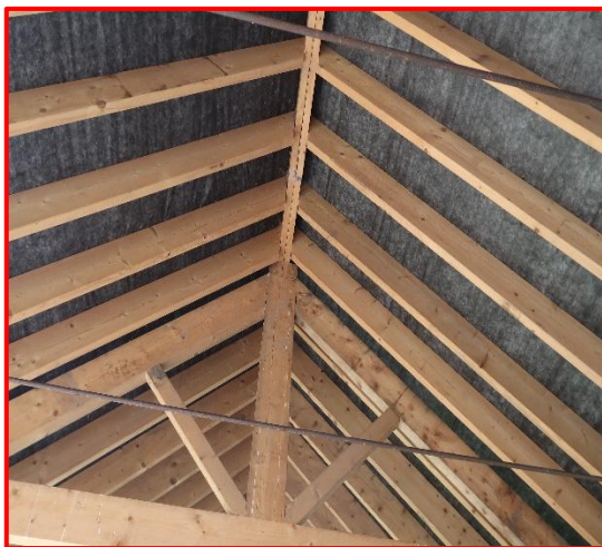
Internal view of barn
