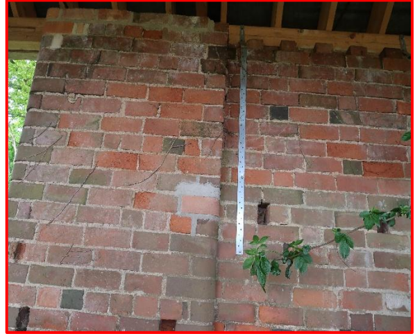
Internal view of barn
