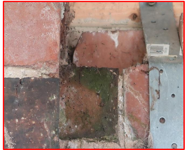
Internal view of barn
