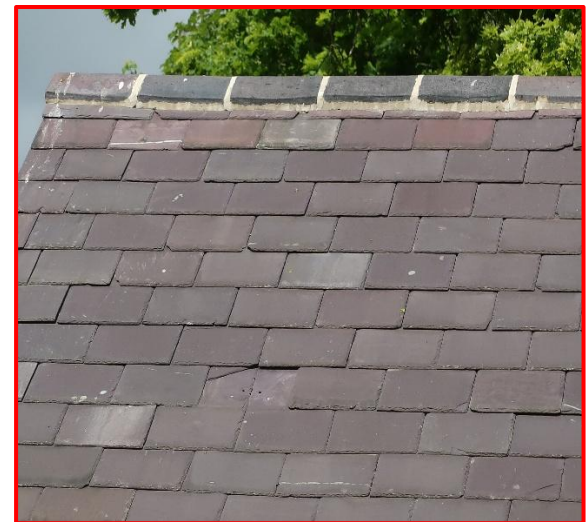
View of barn slate roof
