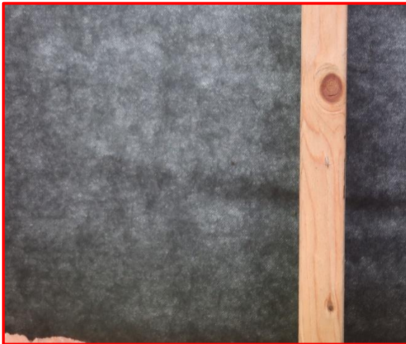
Internal view of barn roof - felt
