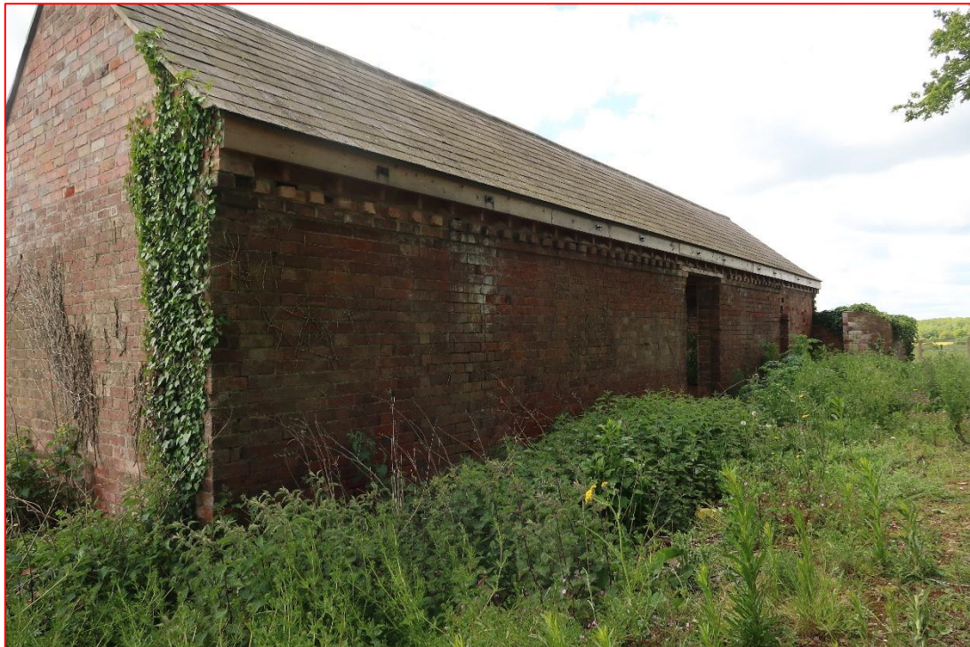
Fig. 1: View of barn.
