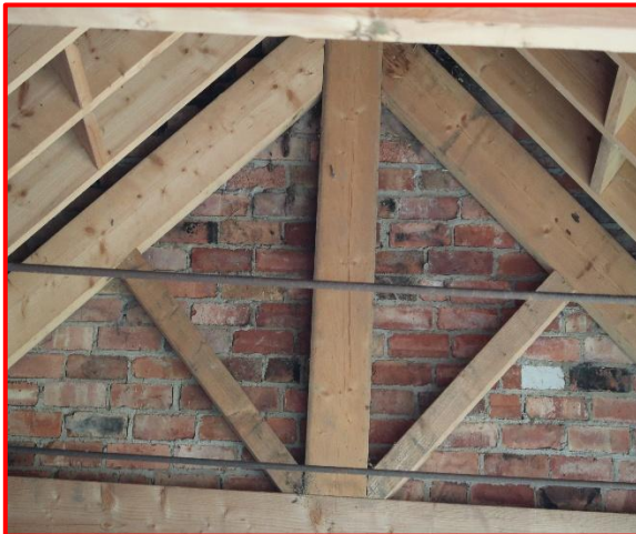
Internal view of barn
