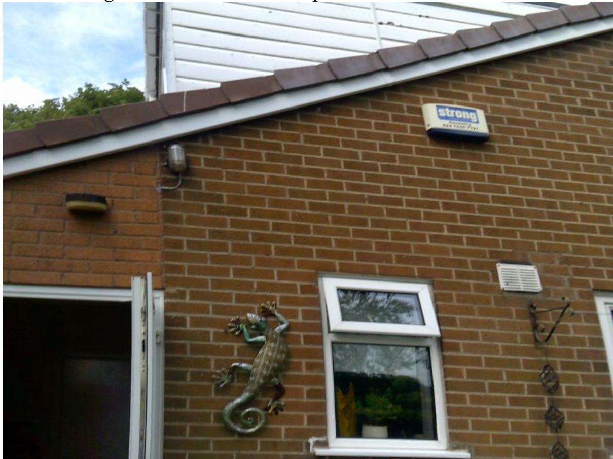
External images of house UPVC endcaps to roof ends
