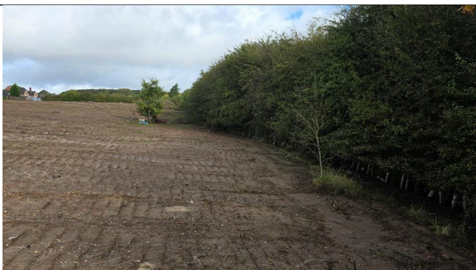
Plate 3: Image showing the site clearance and retained line of trees
