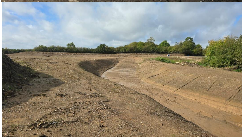
Plate 4: Image showing the site clearance.
