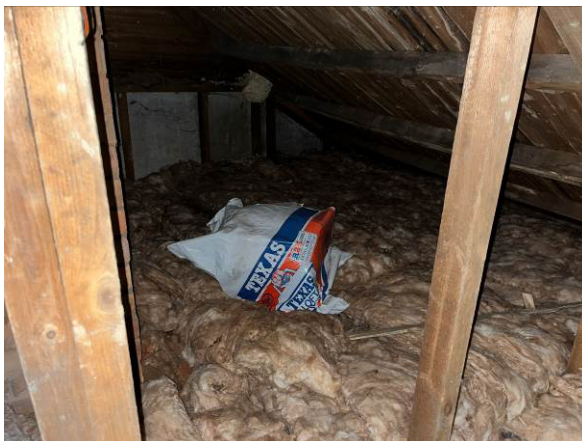
Loft interior south end
