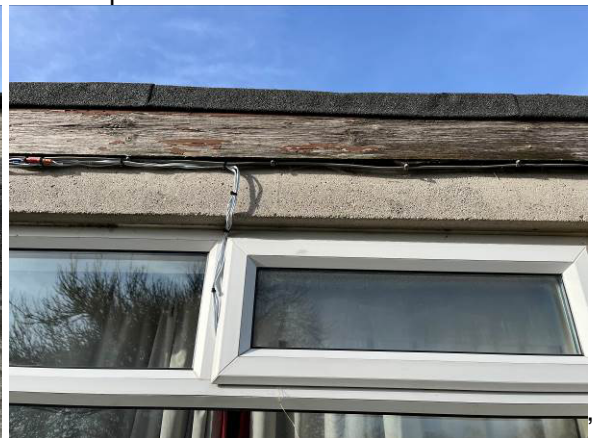
Close up of flat felted roof edge
