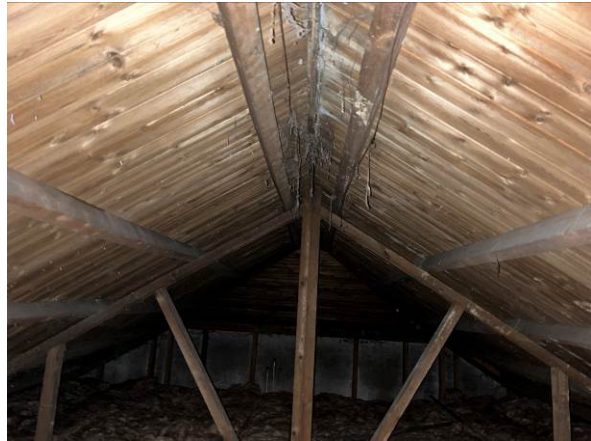
Underside of boarded roof
