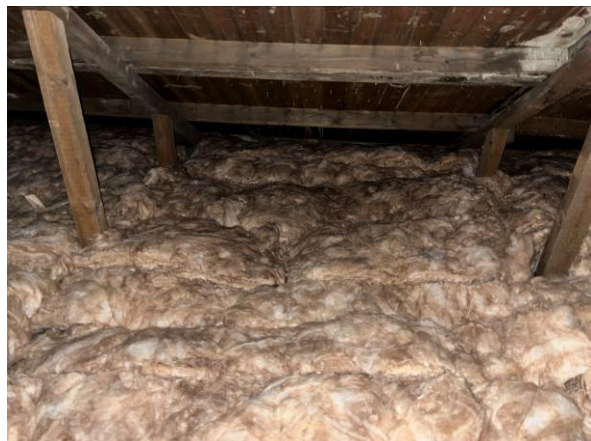
Loft interior and roof edge
