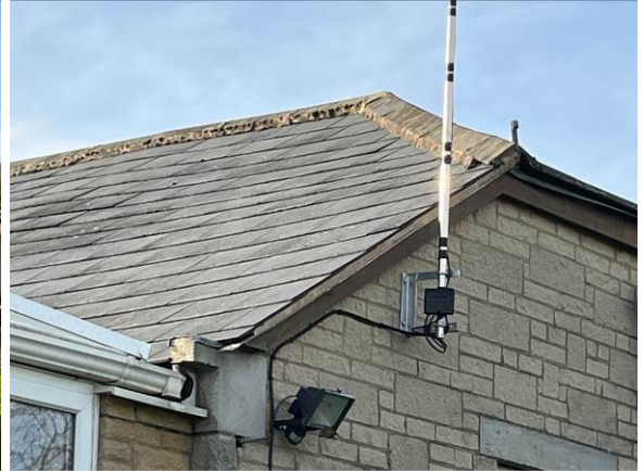
Close up of roof
