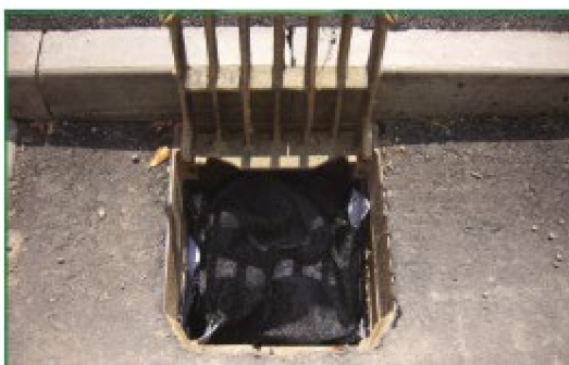
5. Close gully grid.
