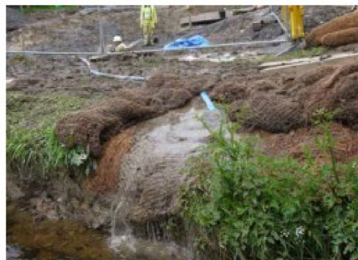
Deployed to treat muddy excavation water
