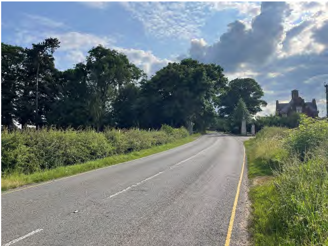
Plate 2 Looking west along The Park/Bosworth Road
