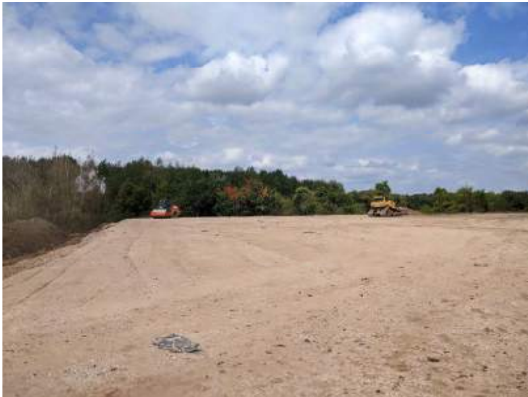
Photo 5: Further build up of Unit 2 levels achieved
