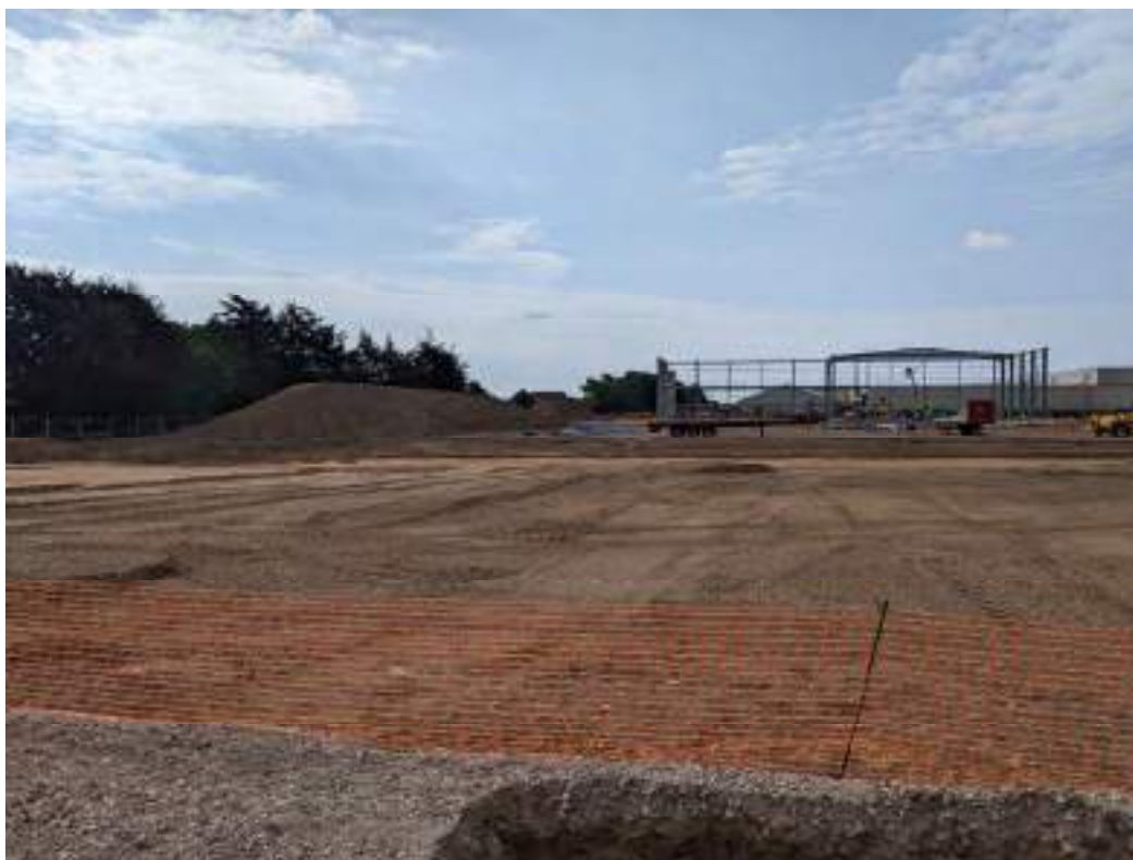
Photo 4: Unit 2 pad foundation excavations to the north of the PAH impacted soils
