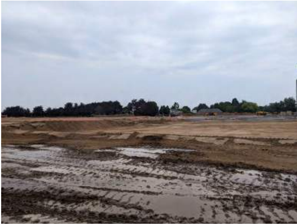
Photo 1: Initial strip of Phase 1 complete
