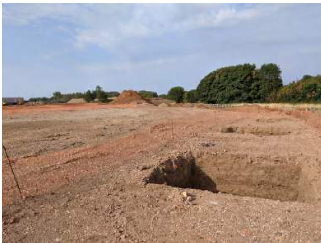
Photo 4: Unit 2 pad foundation excavations to the north of the PAH impacted soils
