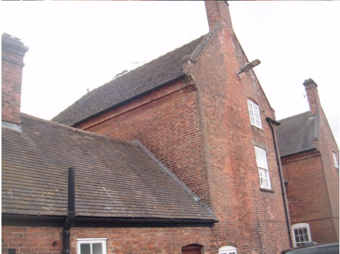
Mani house: single storey section
