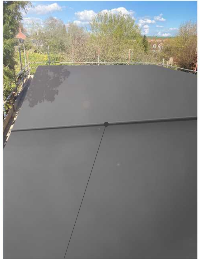
Flat Roof Finish Trim to Joint Line
