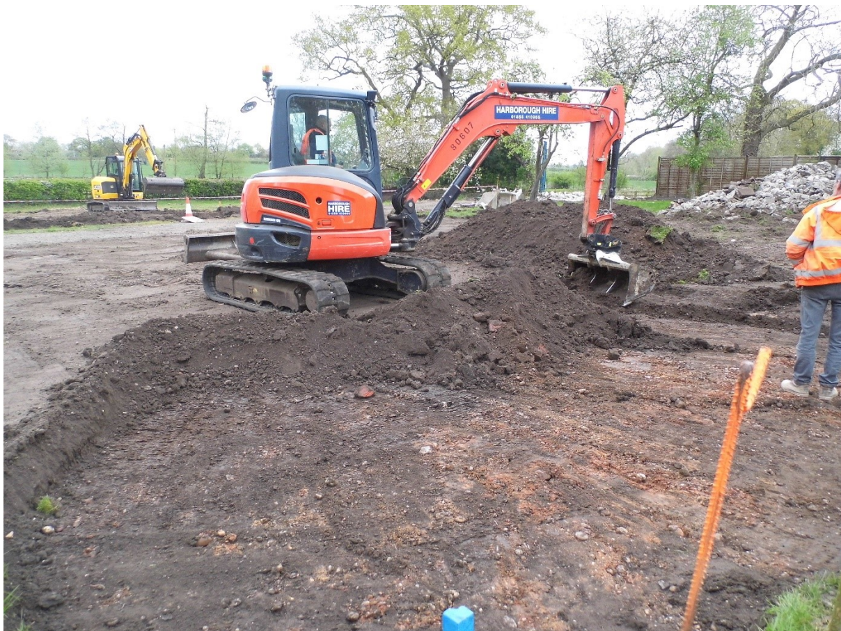
Figure 4: Stripping the topsoil from the southern building plot (looking north).
