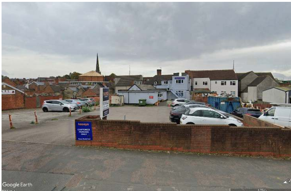
Rear elevation from Trinity Lane
