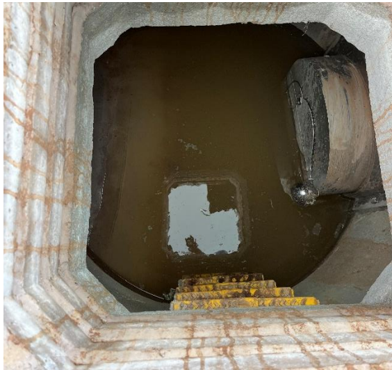
Internal view for new drainage pipework installed
