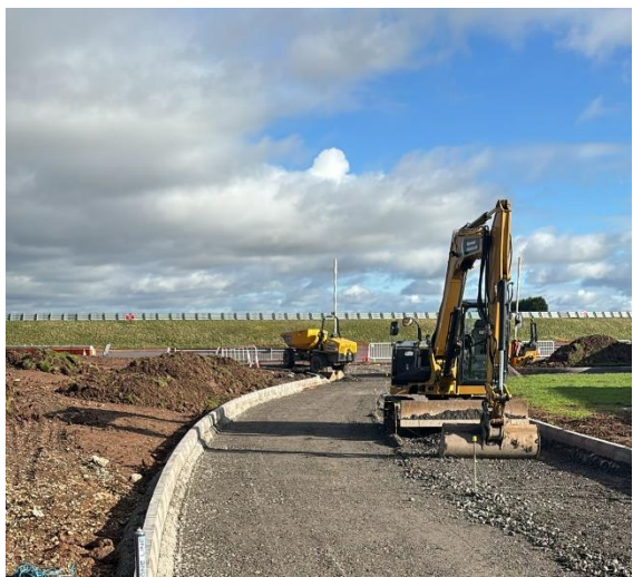
Placement of imported Type 1 for road build up
