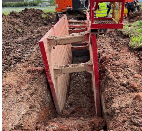
Trench boxing to support installation of new drainage infrastructure
