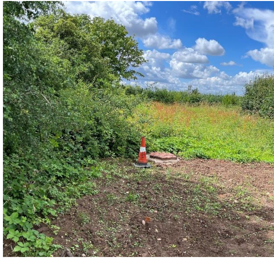
General site conditions ahead of works commencement
