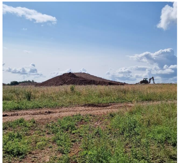
Stockpiling of soils excavated for attenuation ponds
