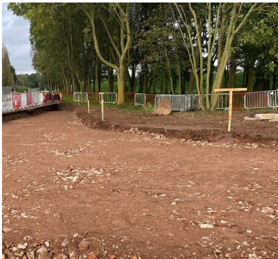
Placement of crushed demolition material to support new roadways
