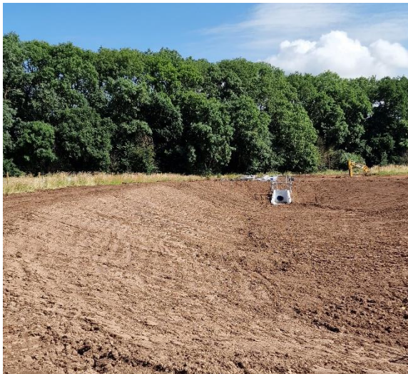
Attenuation pond with new outfall
