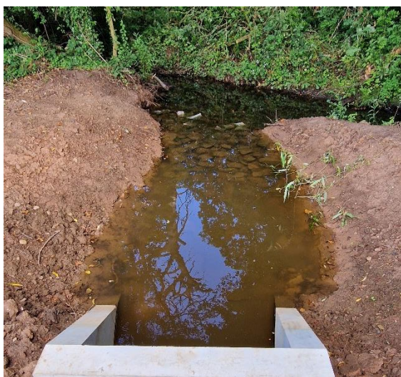
Drainage connection to surrounding ditches
