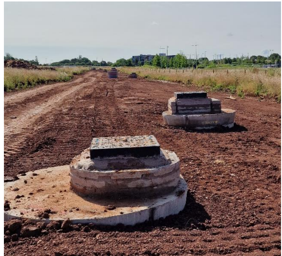
Installation of drainage covers
