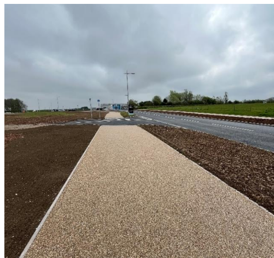
New roadway interchange and footpath installed
