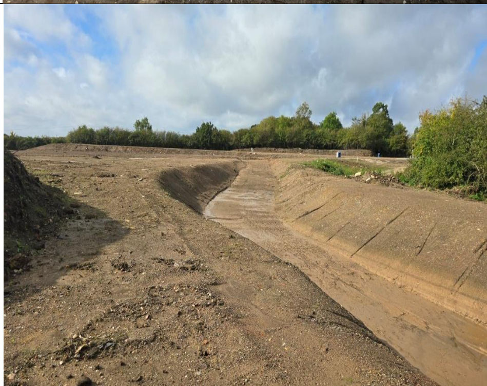
Plate 4: Image showing the site clearance.
