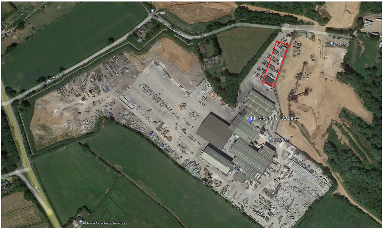
Figure 2 – Google Earth Image showing red line site area
