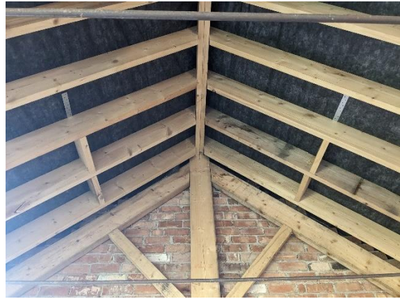
Figure 6- Rafters and membrane
