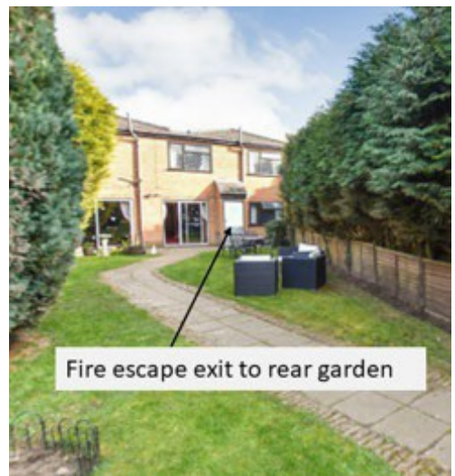
Fire escape exit
