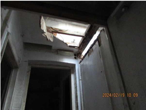
Damage to flat roof
