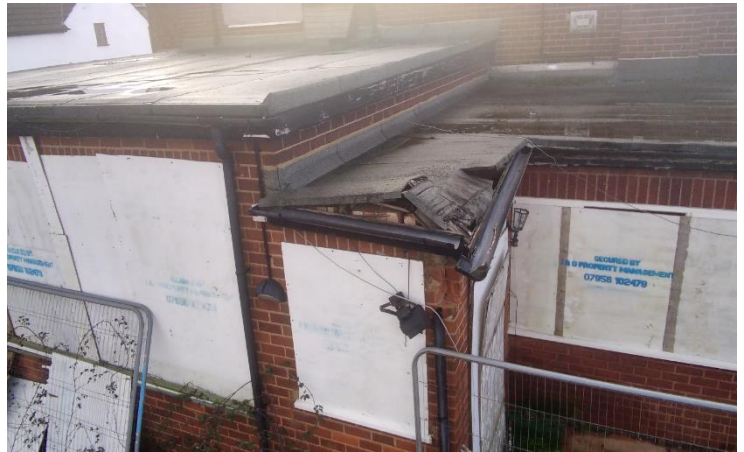
Damage to flat roof
