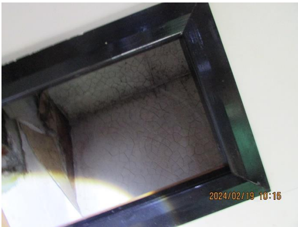
Small roof void with sarking
