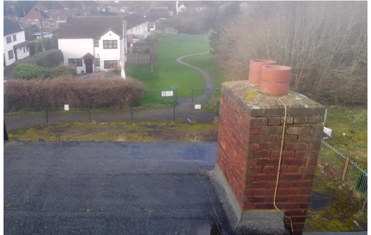
Gaps in brick chimney – Aerial view
