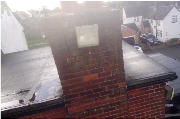
Gaps in brick chimney – Aerial view
