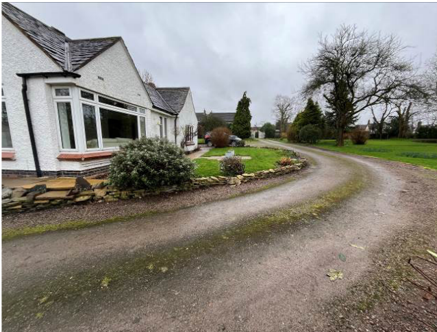
Working area: west corner and side of house
